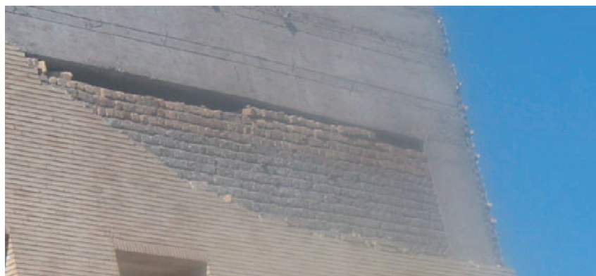
Fig. 7. Solid brick masonry walls in the Bam telephone center building.
