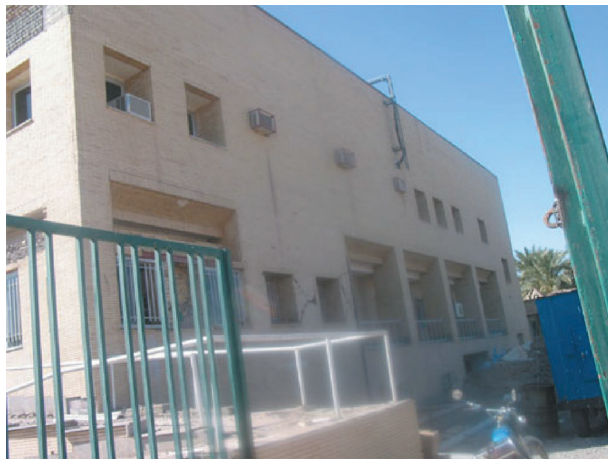
Fig. 2. Bam telephone center RC building after Dec. 2003 Earthquake, North side.
