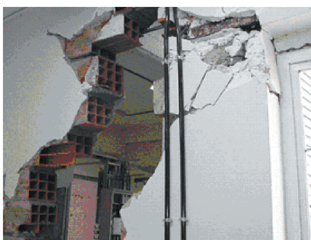
Fig. 8. Hollow block walls in the Bam telephone center building.
