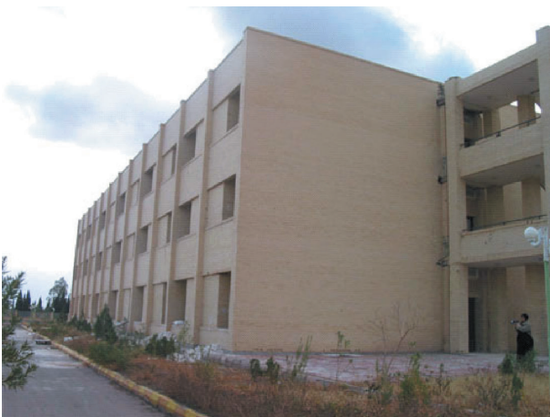
Fig. 23. Bam Azadi hotel which had no structural damage (about 2000 m SW of the strong motion station).
