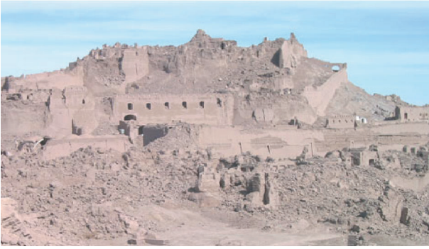
Fig. 10. Arg-e-Bam, example of adobe structure (Ad type).
