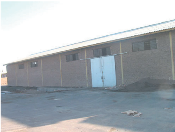
Fig. 16. Special steel frame-masonry structures, M-S-F type.
