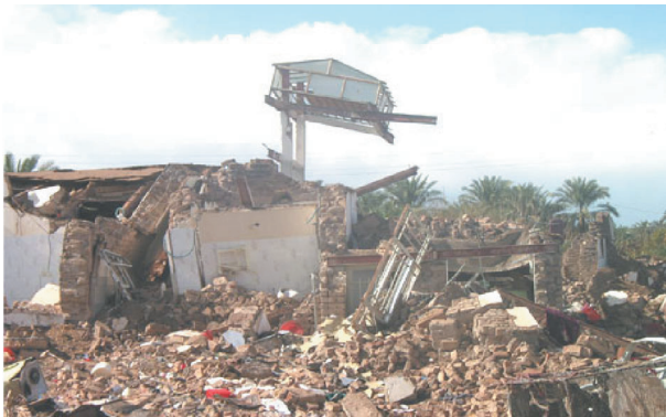
Fig. 11. Masonry Buildings in Bam, M Type.
