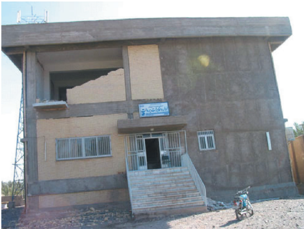
Fig. 22. Baravat village telephone center, which had no structural damage.
