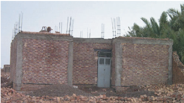
Fig. 12. Reinforced Masonry Buildings in Bam, M-C Type.
