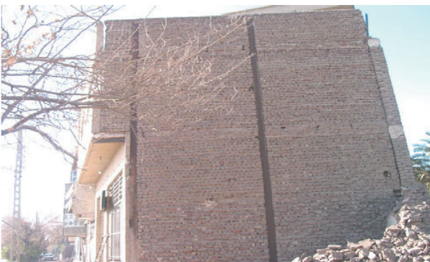
Fig. 13. Masonry with steel frame buildings, M-S type.
