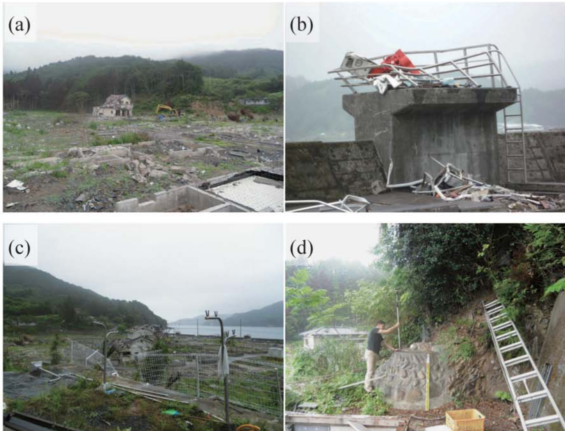
Fig. A204. (a)-(c) Damage at Ogatsucho-Myojin. (d) Tsunami trace survey point behind Namikirifudo (a Buddhist statue) at the northern slope (M56).
