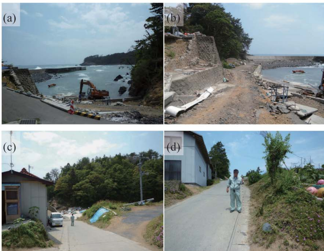
Fig. A158. (a)-(c) Damage at Utatsu-Hiradana. (d) Tsunami trace survey point at a slope beside Mr. Sato's house (M24).
