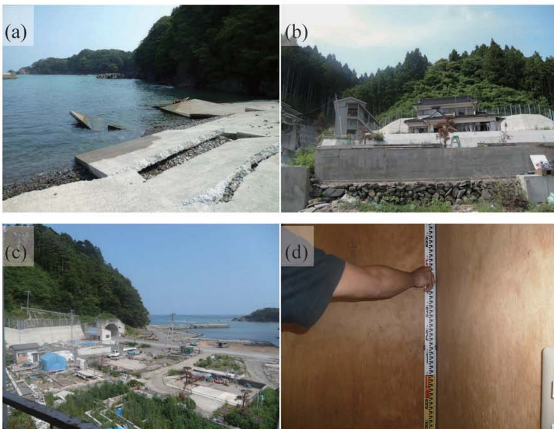
Fig. A180. (a)-(c) Damage at Kozashi. (d) Tsunami trace survey point on a wall of a house (1.15m above the second floor, M38)
