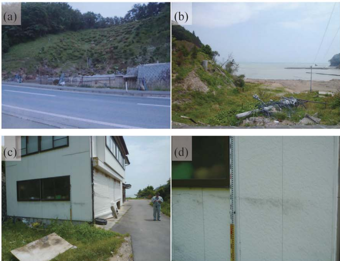
Fig. A152. (a)-(b) Damage at Motoyoshicho-Nijuichihama. (c)-(d) Tsunami trace survey point on a wall of Mr. Oikawa's house (1.27 m above ground level, M13).
