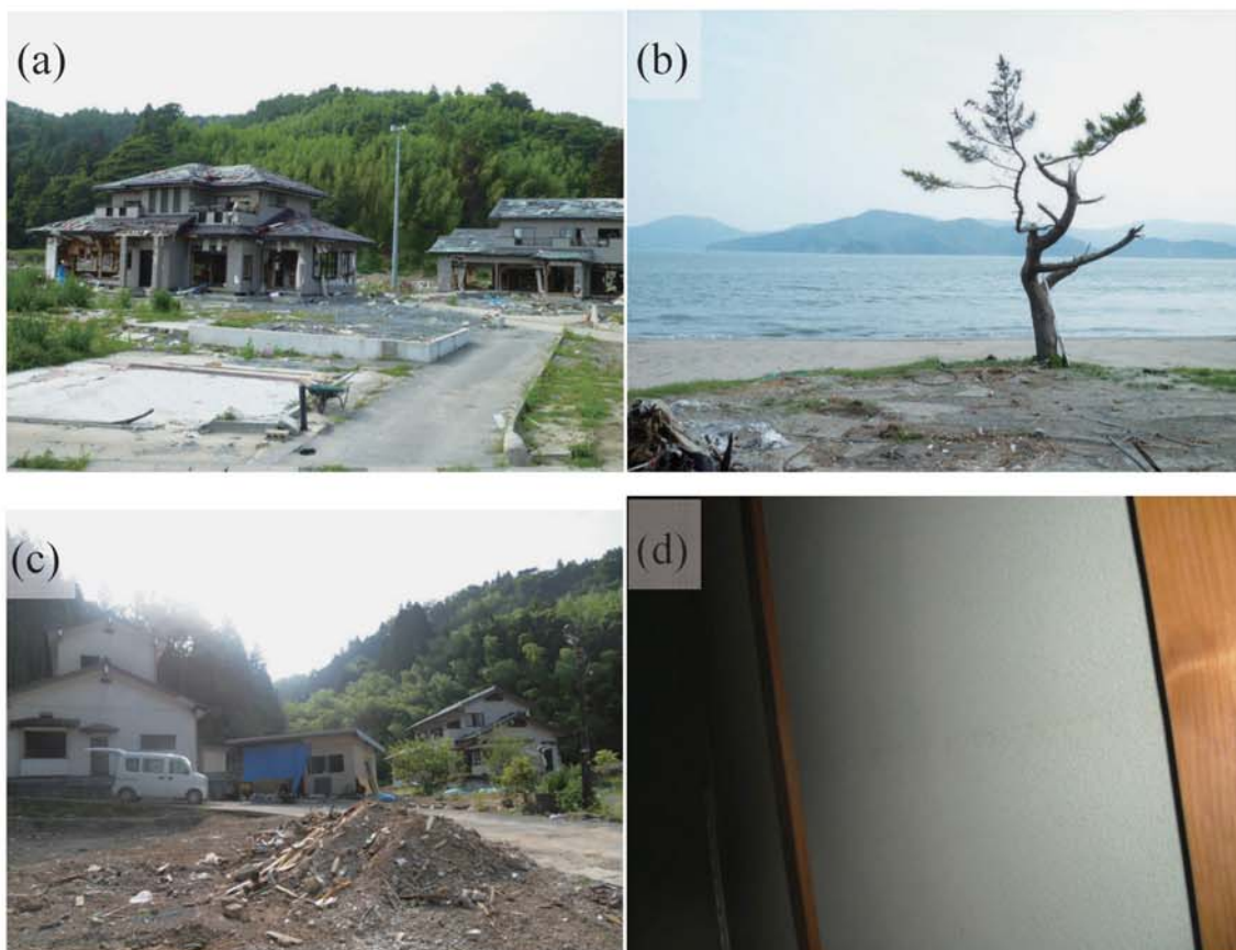
Fig. A188. (a)-(c) Damage at Shirahama. (d) Tsunami trace survey point on a wall of the second floor of Mr. Sato's house (6.09 m above ground level, M42).
