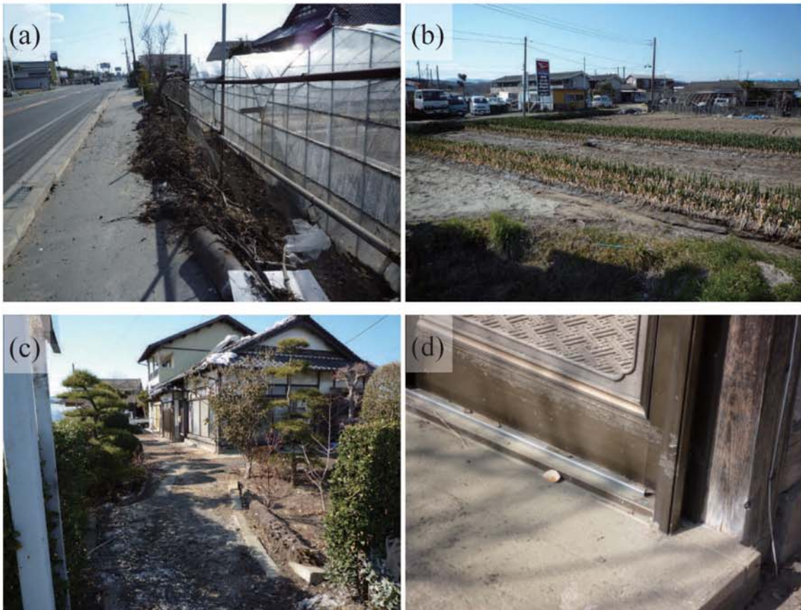
Fig. A244. (a) Debris on the roadside of the National Highway 6 in Sekinamicho-kamiokashimo. (b) Sand deposit and dead farm products in a field at Sekinamicho-Kamiokashimo. (c) Mr. Aida's house at Sekinamicho-Kamiokashimo (tsunami trace survey point). (d) Watermark at the lower part of entrance sliding doors of Mr. Aida's house (0.15 m above ground level, B7).
