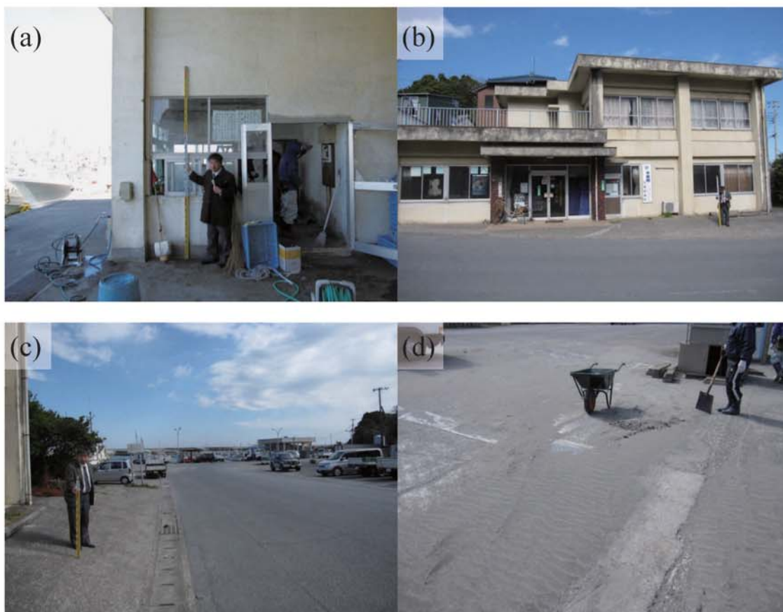
Fig. A322. (a) Watermark on windowpanes of fishery market office building (2.15 m above ground level; C20) (b)-(c) Tsunami inundation limit at a slope in front of the Isumitobu fishery association building (Taito affiliate)(C21). (d) Sand deposit carried by the tsunami in Taito Fishing Port.
