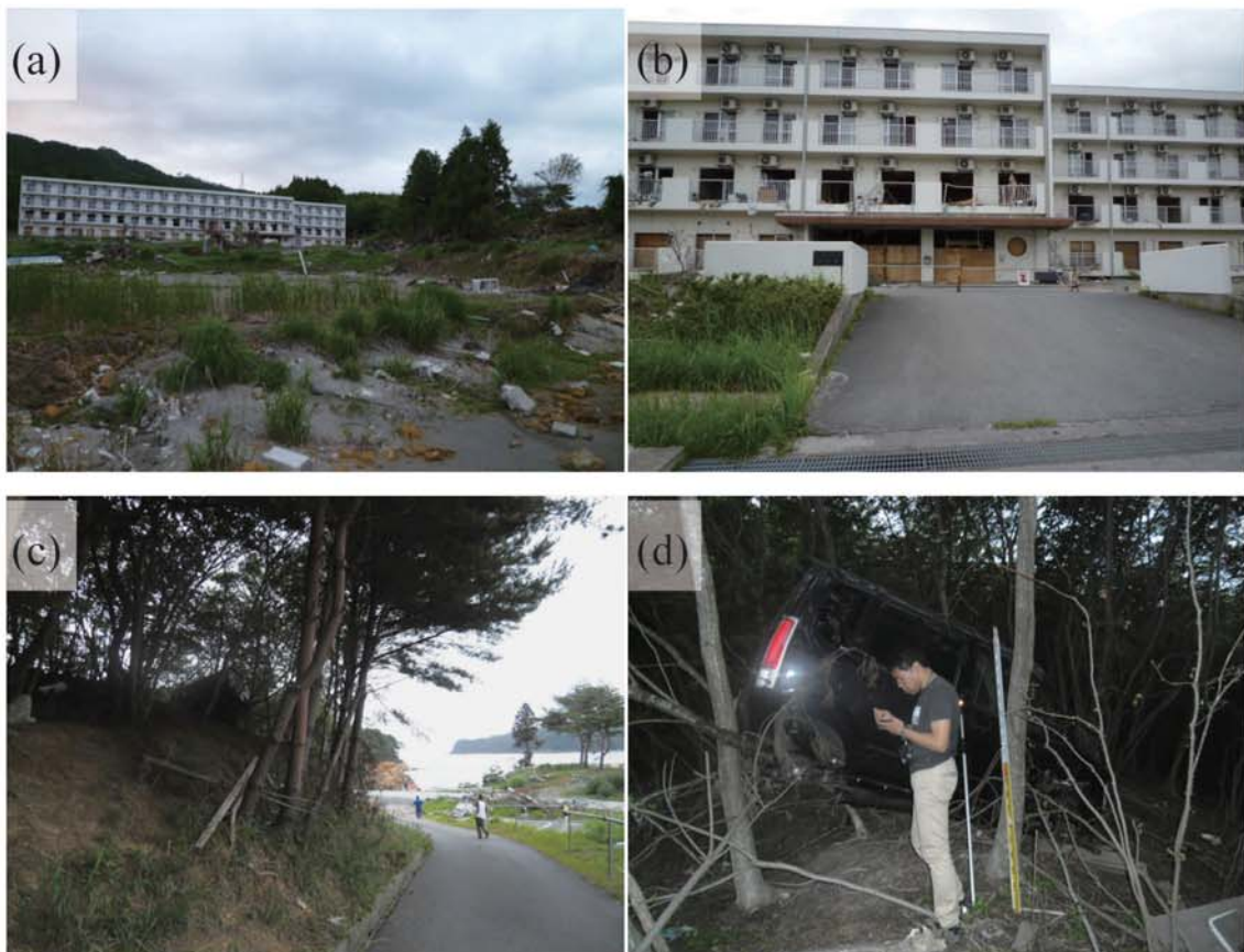
Fig. A220. (a)-(b) Damage at Samenoura. (c)-(d) Tsunami trace survey point on a hill behind the Samenoura dormitory of Tohoku Electric Power Engineering (1.10 m above ground level, M65).
