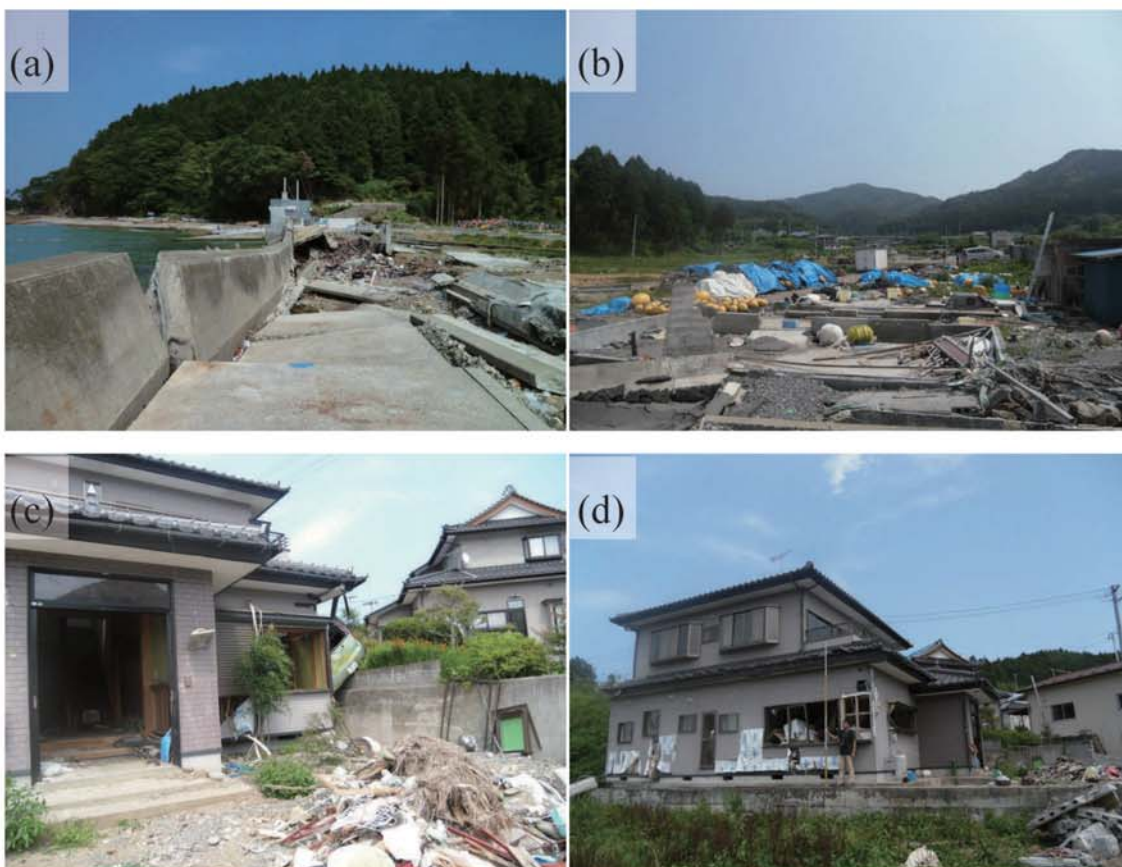
Fig. A176. (a)-(c) Damage at Takihama. (d) Tsunami trace survey point on the roof of a house (2.75 m above ground level, M36).
