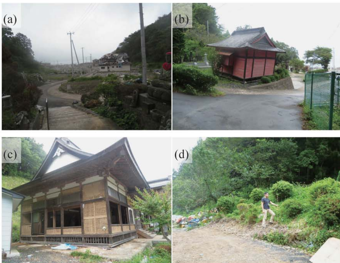
Fig. A210. (a)-(c) Damage at Wakehama. (d) Tsunami trace survey point on a slope beside the Kogenin (M59).
