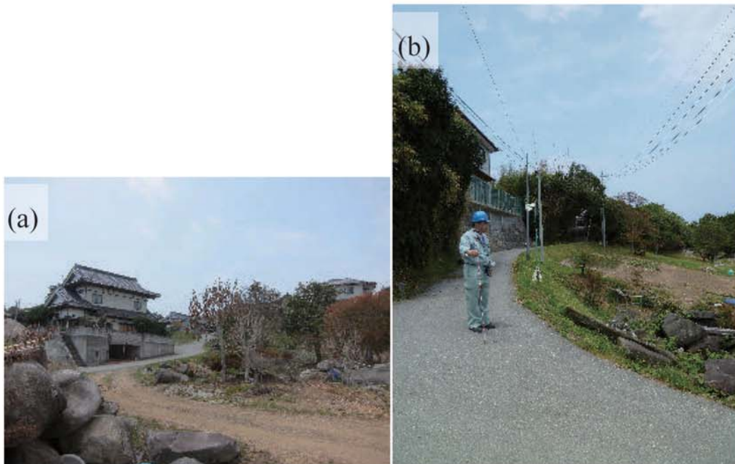
Fig. A134. (a) Damage at Karakuwacho-Baba. (b) Tsunami trace survey point at the southern slope (M1).
