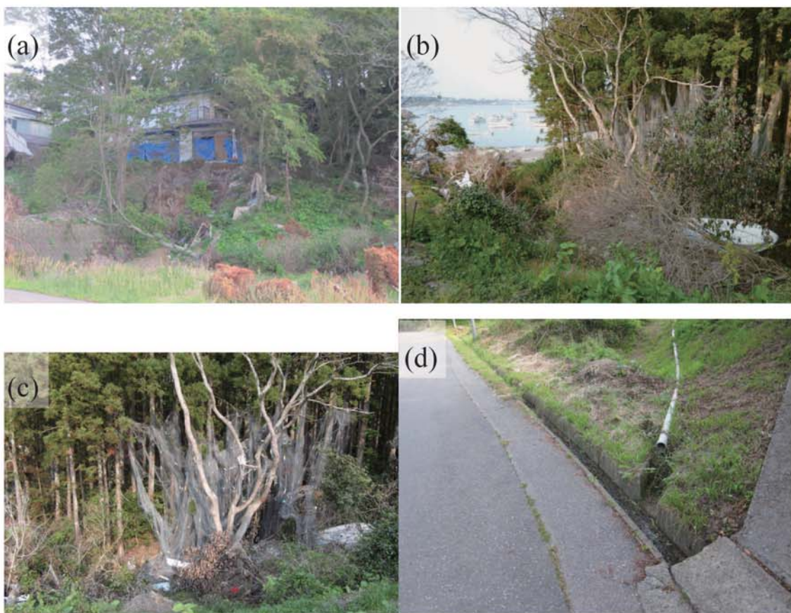
Fig. A146. (a)-(c) Damage at Motoyoshicho-Amagasawa (Hikado Fishing Port). (d) Tsunami trace survey point on a slope (M10).
