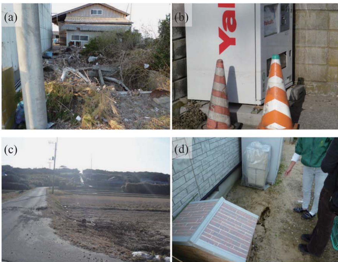
Fig. A286. (a) Debris carried by the tsunami in Takeigama. (b) Watermark on a side of a vending machine beside the fisheries processing factory (0.495 m above ground level, B32). (c) Tsunami inundation limit on a road in Takeigama (B33). (d) Watermark on a side of a foundation of Mr. Kudo's house in Hamatsuga (0.08 m above ground level, B34).
