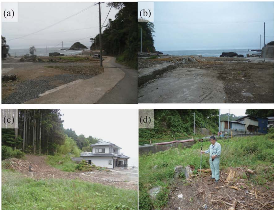
Fig. A198. (a)-(c) Damage at Ogatsucho-Osu. (d) Tsunami trace survey point on the slope (M52).
