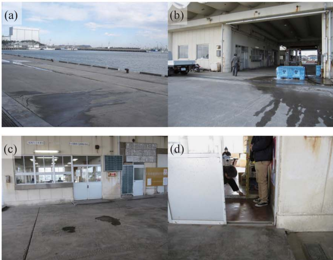
Fig. A324. (a)-(c) Ohara Fishing Port. (d) Tsunami trace survey point at the entrance of Isunitobu fishery association office (C22).
