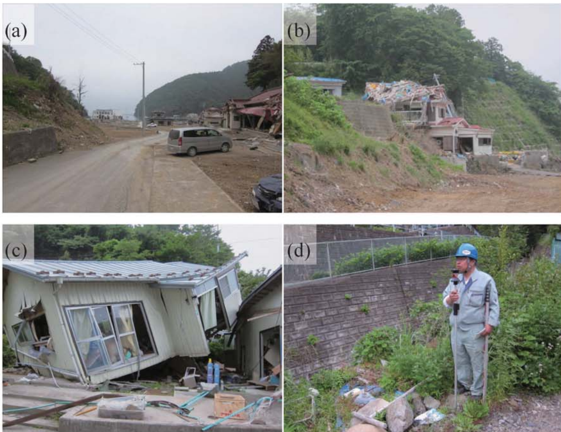
Fig. A196. (a)-(c) Damage at Ogatsucho-Funakoshi. (d) Tsunami trace survey point on a southern slope beside a grave (M51).
