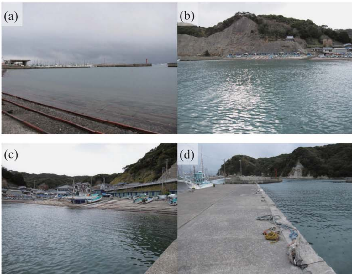
Fig. A332. (a)-(c) Hamanamegawa Fishing Port. (d) Tsunami trace survey point at the top of a quay (C28).
