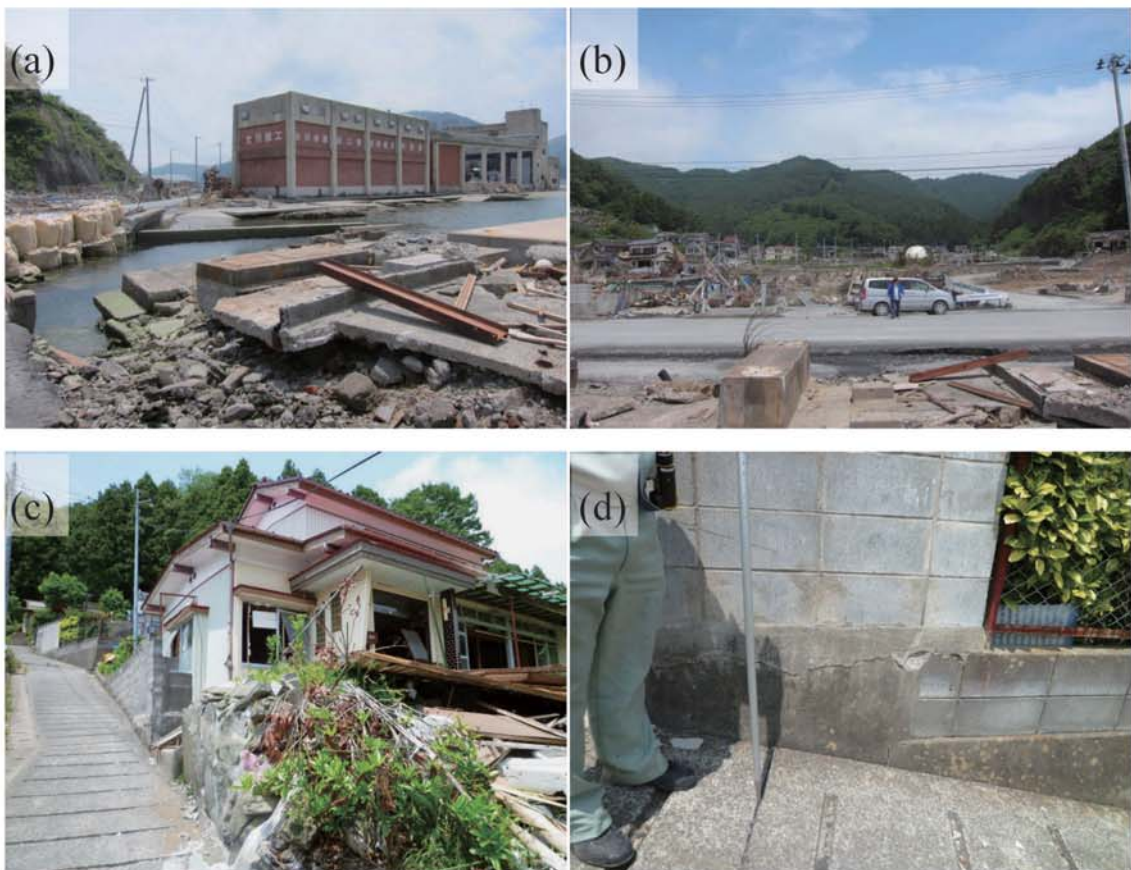
Fig. A214. (a)-(b) Damage at Ishihama. (c)-(d) Tsunami trace survey point at a slope beside the entrance to a grave site (M61).
