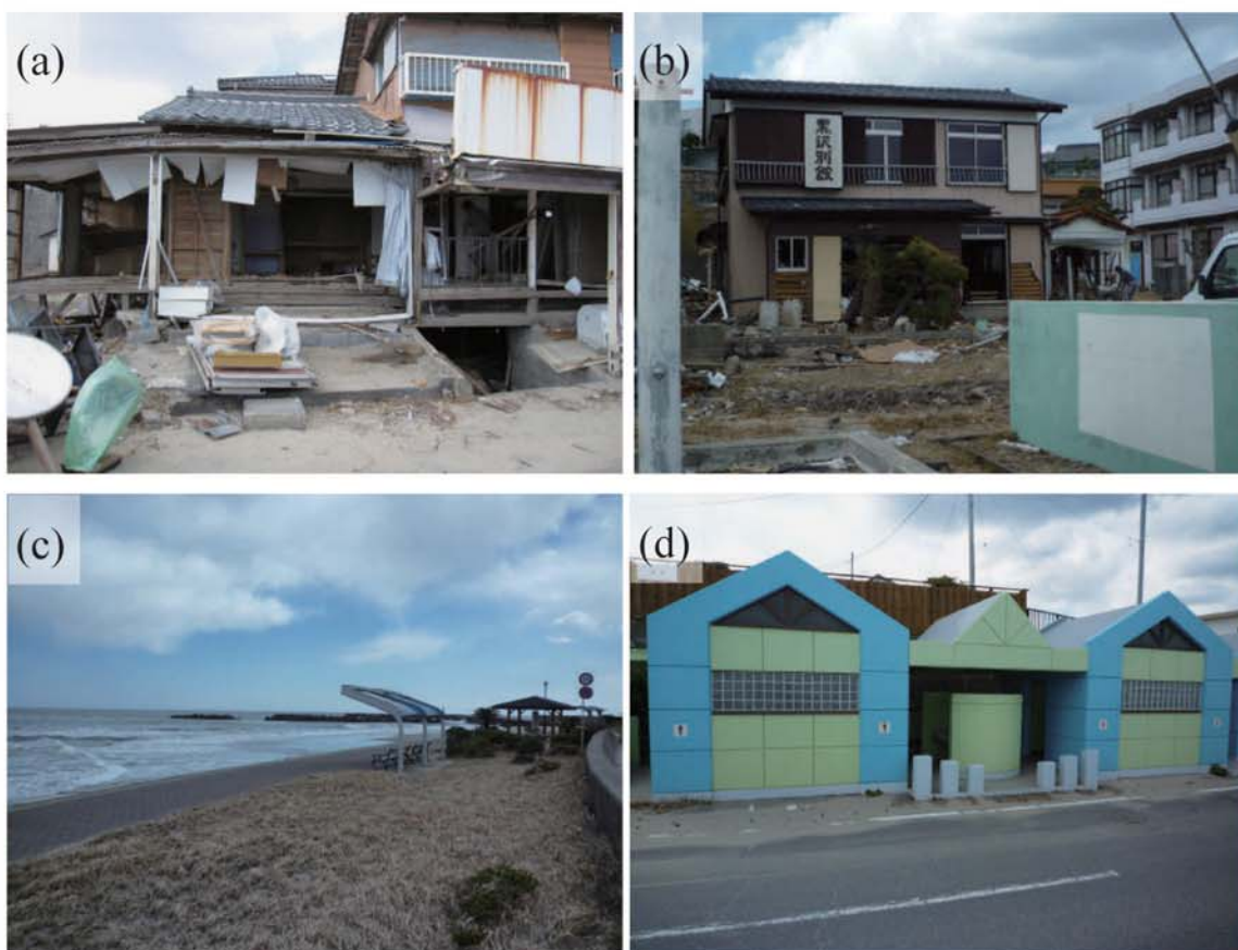
Fig. A270. (a)-(b) Damage at Kawaragocho. (c) Kawarago Beach. (d) Public lavatory beside Kawarago Beach (tsunami trace survey point). (e) Watermark on an inner wall of the public lavatory (0.55 m above ground level, B22). (f) Kawarago Fishing Port. (g) Building of the fishery association in Kawarago Fishing Port (tsunami trace survey point). (h) Watermark on an inner wall at the first floor of the fishery association building (2.035 m above the floor level, B23).
