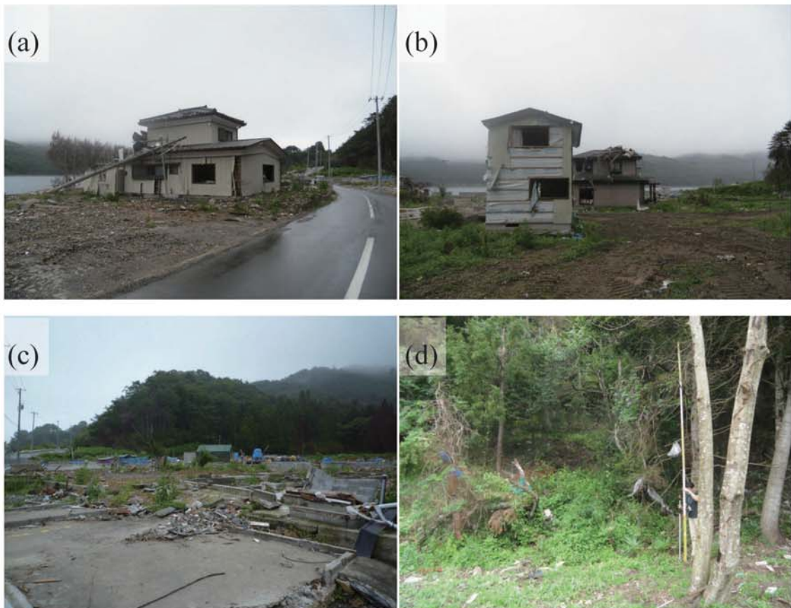
Fig. A208. (a)-(c) Damage at Karakuwa. (d) Tsunami trace survey point on the southern slope (4.90 m above ground level, M58).
