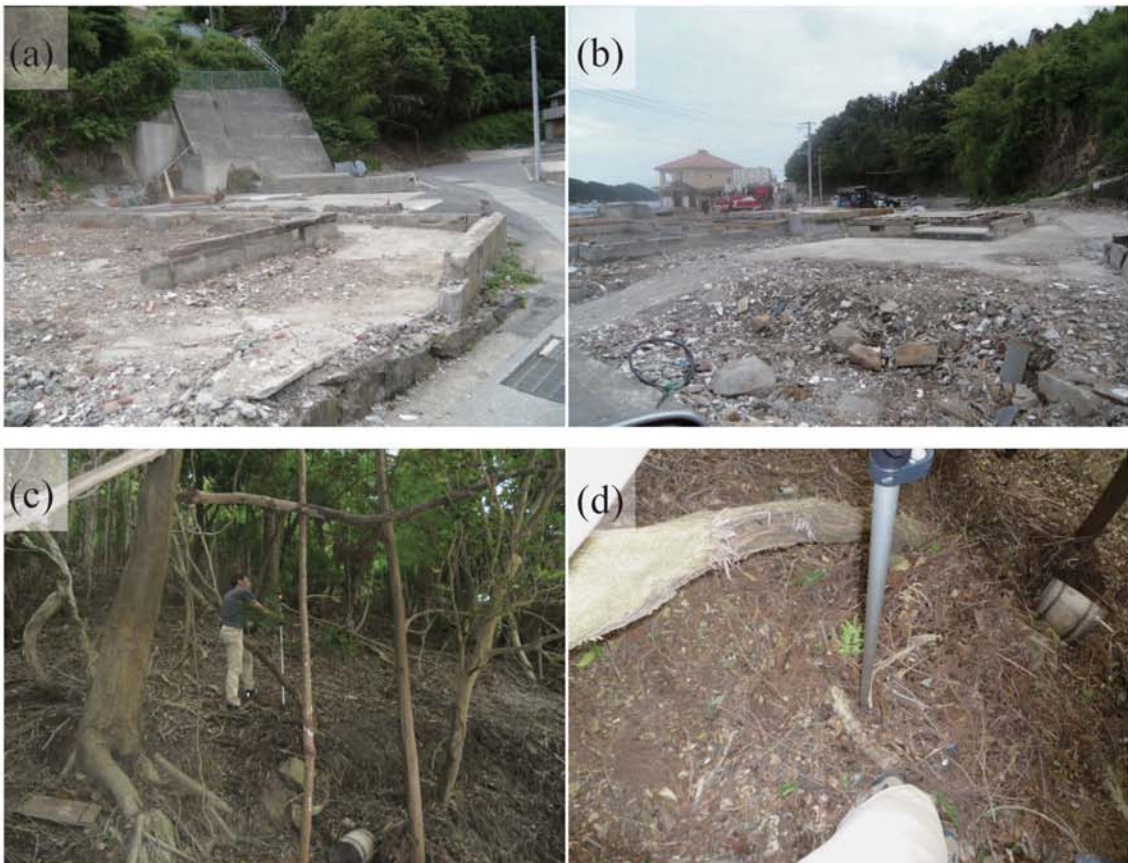
Fig. A232. (a)-(b) Damage at Fukkiura. (c)-(d) Tsunami trace survey point at an eastern slope (M73).
