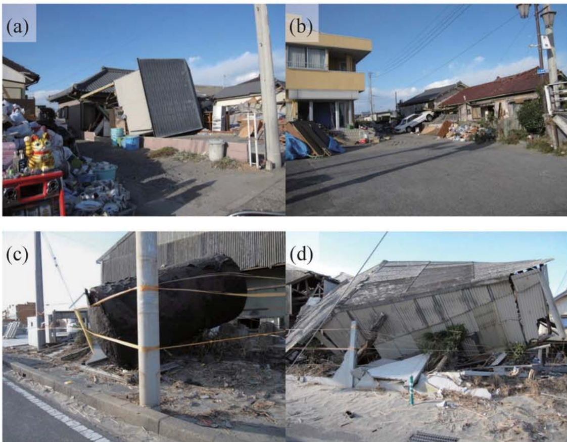
Fig. A298. (a)-(j) Damage at Hiramatsu.
