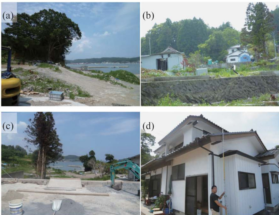
Fig. A172. (a)-(c) Damage at Shizugawa-Hayashi. (d) Tsunami trace survey point on a wall of Mr.Watanabe's house (Testimony of an inhabitant, 3.55 m above ground level, M34).
