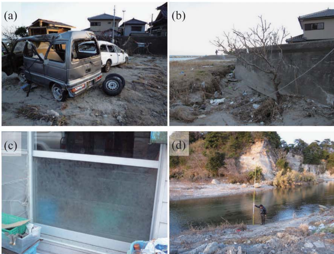
Fig. A256. (a)-(b) Damage near the mouth of the Juo River in Kawajiricho. (c) Watermark on windowpanes of Mr. Suzuki's house (1.04 m above ground level, B13). (d) Measuring ground height at the survey point based on the water surface of the Juo River.
