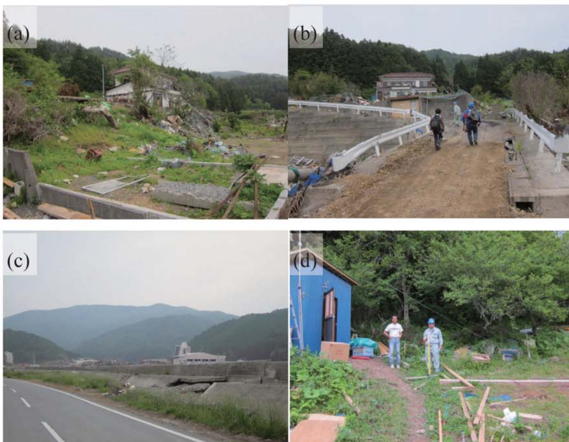
Fig. A206. (a)-(c) Damage at Funatoshinmei. (d) Tsunami trace survey point at a slope behind Mr. Sugiyama's house (M57).
