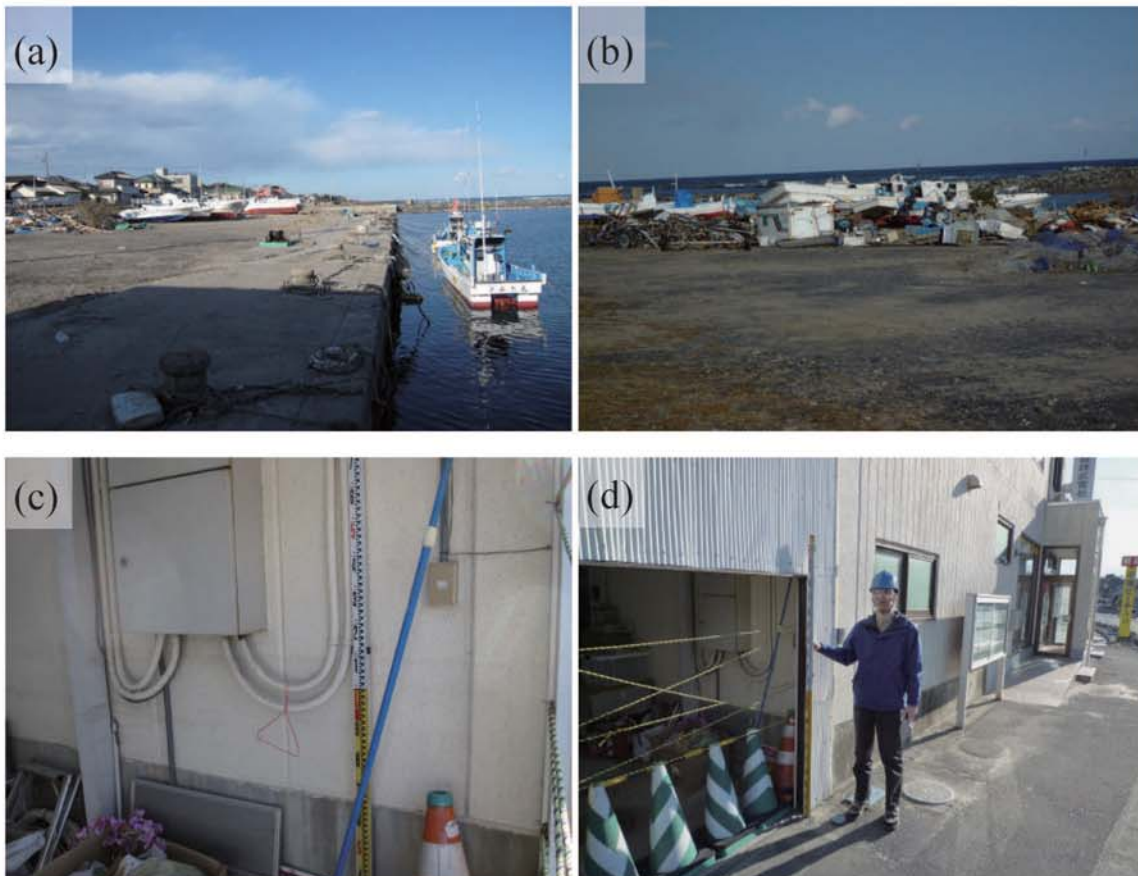
Fig. A280. (a)-(b) Damage at Hiraiso Fishing Port. (c)-(d) Watermark on a wall of a building behind the port (1.085 m above ground level, B28).
