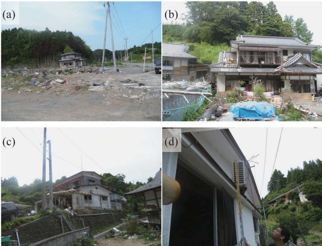
Fig. A186. (a)-(c) Damage at Omuro. (d) Tsunami trace survey point at an outdoor unit of an air conditioner on an eave of Mr. Sasaki's house (2.75 m above ground level, M41)
