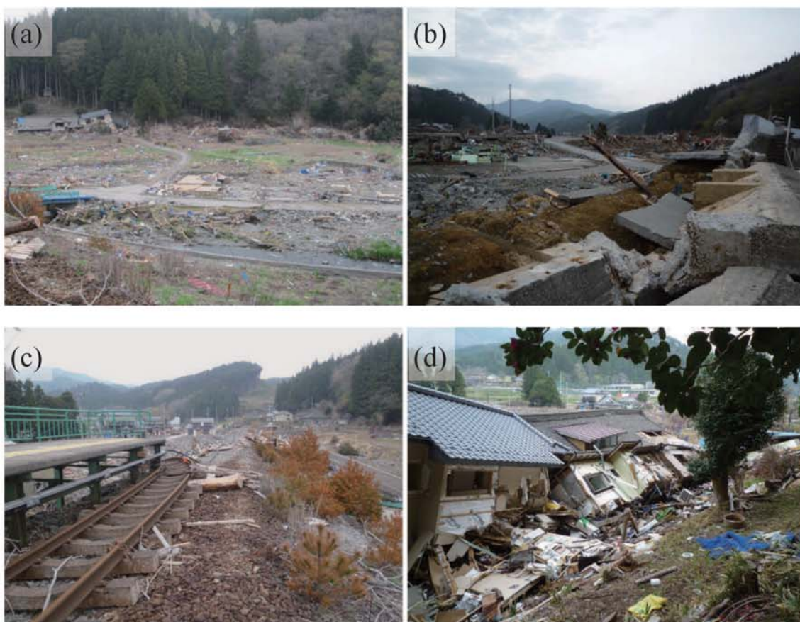
Fig. A126. (a)-(d) Damage at Horei. (e) Tsunami inundation limit on the northeastern slope at Horei station (I130). (f) Debris piled up around the survey point of I130. (g)-(h) Tsunami inundation limit at a field in front of a house (I131). (i)-(j) Tsunami trace survey point on the railroad of the Sanriku railway (I132).
