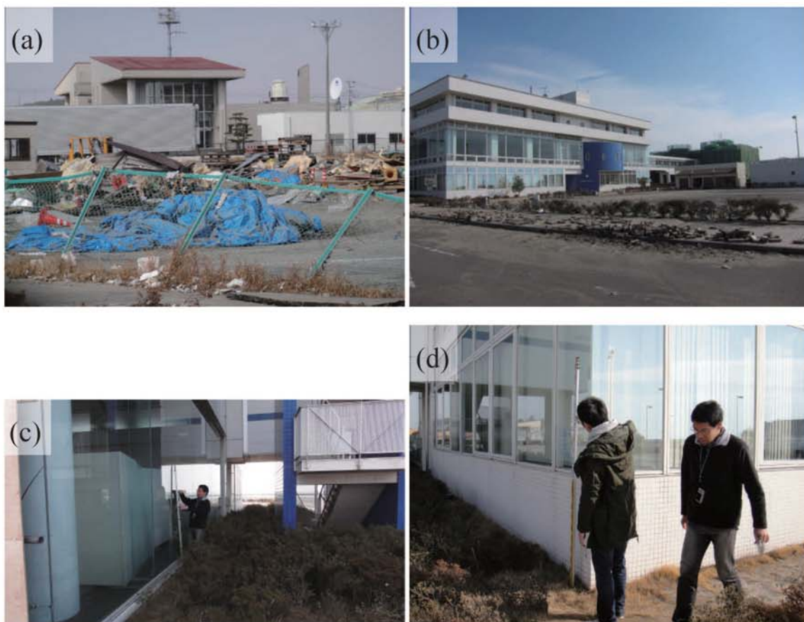
Fig. A284. (a) Damage at Minatocho (Ibaraki Port, Oarai District). (b) Ferry terminal building at Oarai Port. (c) Watermark on windowpanes of ferry terminal building (1.575 m above ground level, B30). (d) Another watermark on windowpanes of the ferry terminal building (1.65 m above ground level, B31).
