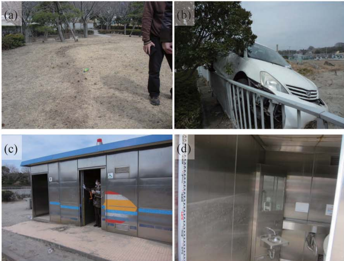
Fig. A274. (a) Trace of tsunami inundation limit on a hill at Nagisa Park. (b) Drifted car that crashed against a fence at Nagisa Park. (c) Public lavatory in Nagisa Park (tsunami trace survey point). (d) Watermark on an inner wall of the public lavatory (1.52 m above ground level, B25).
