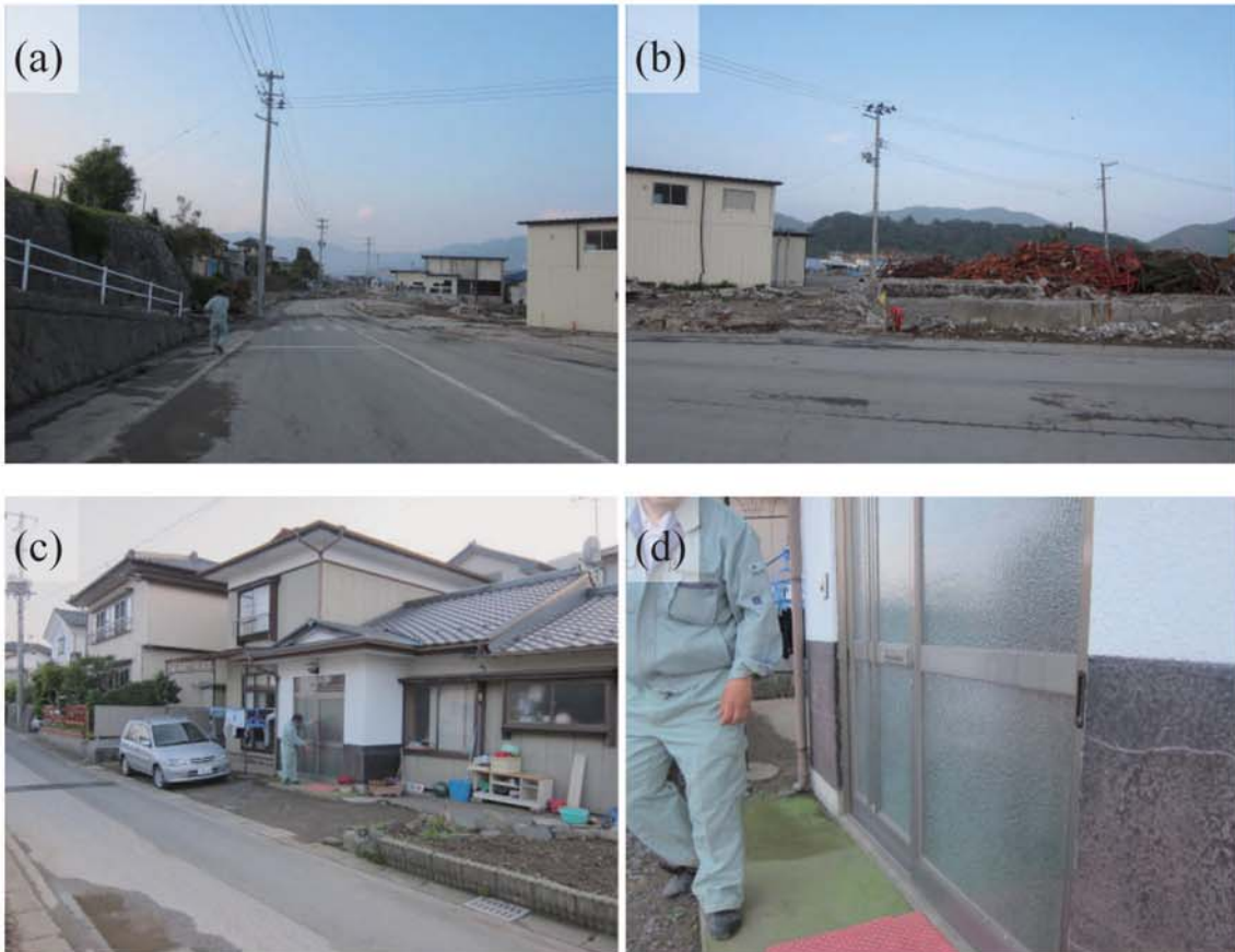
Fig. A130. (a)-(b) Damage at Miyanomae. (c) Mr. Kawahara's house at Miyanomae (tsunami trace survey point). (d) Watermark on the windowpanes of the sliding doors at the entrance of Mr. Kawahara's house (0.7 m above ground level, I135).
