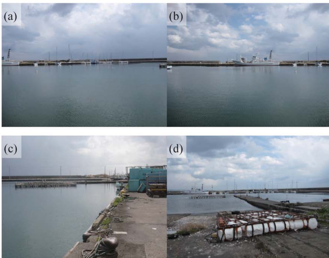
Fig. A346. (a)-(b) Chikura Fishing Port. (c) Quay inundated by the tsunami to a small depth (C37). (d) The other quay with a height equivalent to the Tsunami height at the port (C38).
