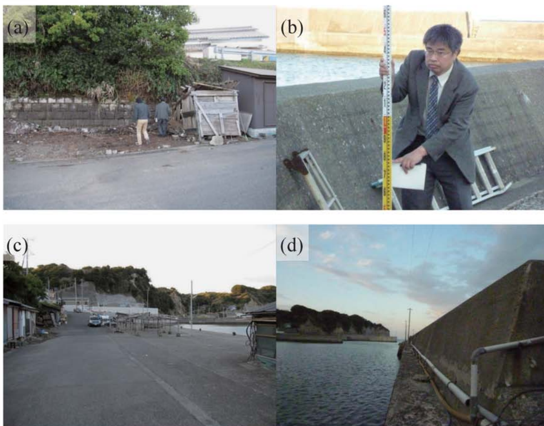
Fig. A326. (a) Damage at Iwafune Fishing Port. (b) Aluminum ladder inundated by the tsunami (C23). (c) Framework of shack inundated by the tsunami (C24). (d) Pipe completely inundated by the tsunami (C25).
