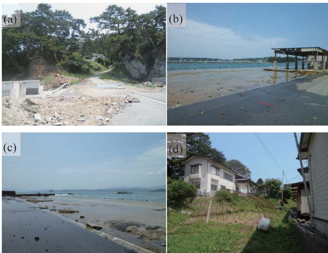
Fig. A162. (a)-(c) Damage at Utatsu-Osaki. (d) Tsunami trace survey point beside a water well near Mr. Iwaishi's house (M26).
