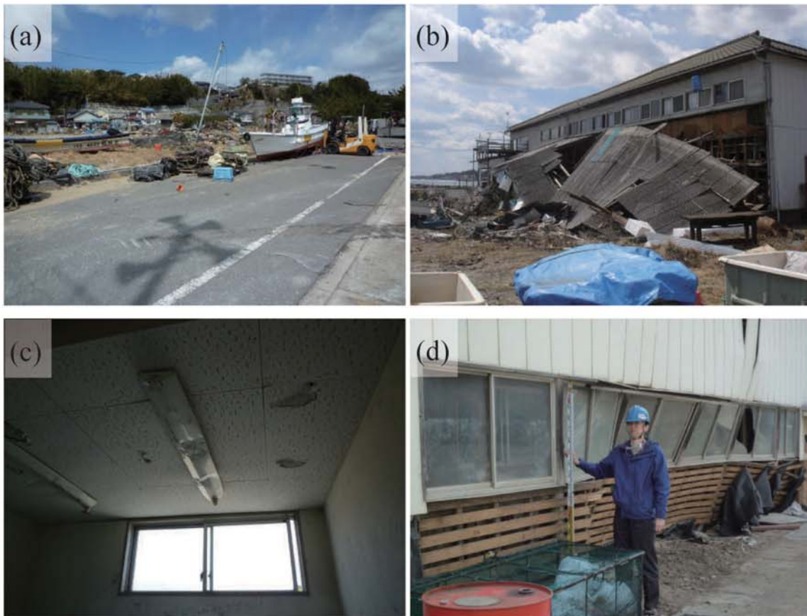
Fig. A266. (a)-(b) Damage at Ose Fishing Port. (c) Tsunami reached the ceiling on the first floor of the fishery association building in Ose Fishing Port. (d) Watermark on windowpanes of warehouse behind the port (1.75 m above ground level, B19).
