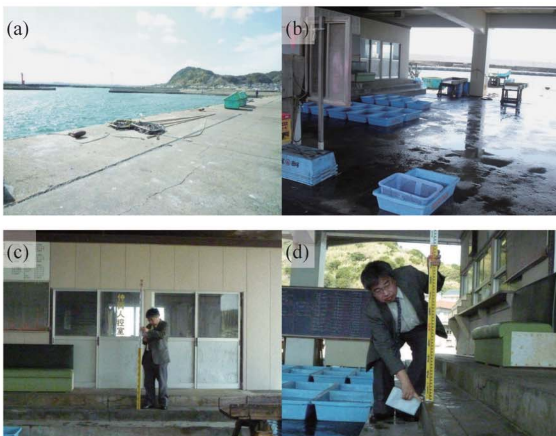
Fig. A342. (a) Wada Fishing Port. (b)-(d) Tsunami trace survey point at the second step of stairs in front of Wada Fishing Port office (C34).
