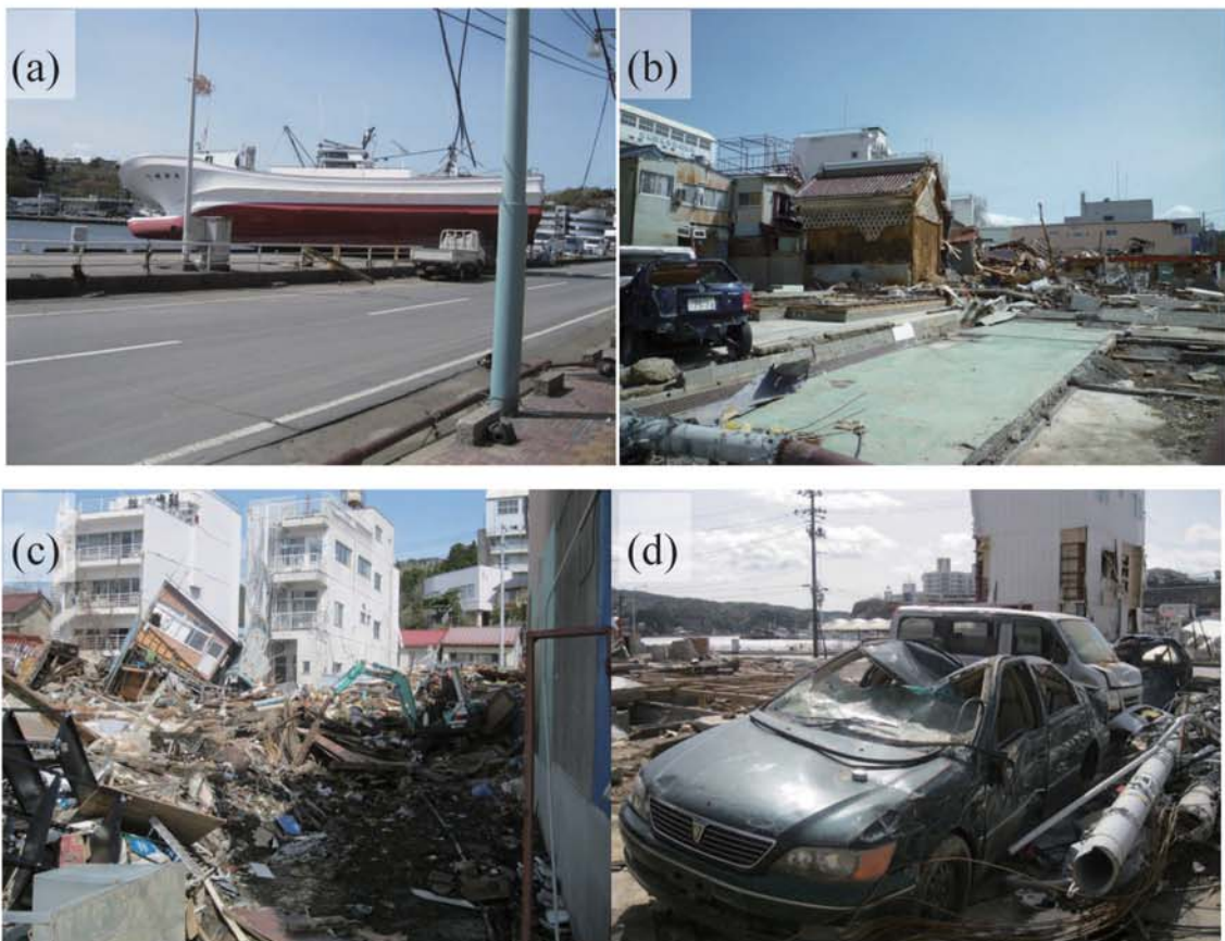
Fig. A142. (a)-(f) Damage at Minamimachikaigan (Kesennuma Port). (g)-(j) Watermark on a wall of the municipal parking and surrounding buildings (2.60 m, 3.12 m, 3.08 m, and 2.95 m above ground level, respectively, M6, M7, M8, M5).
