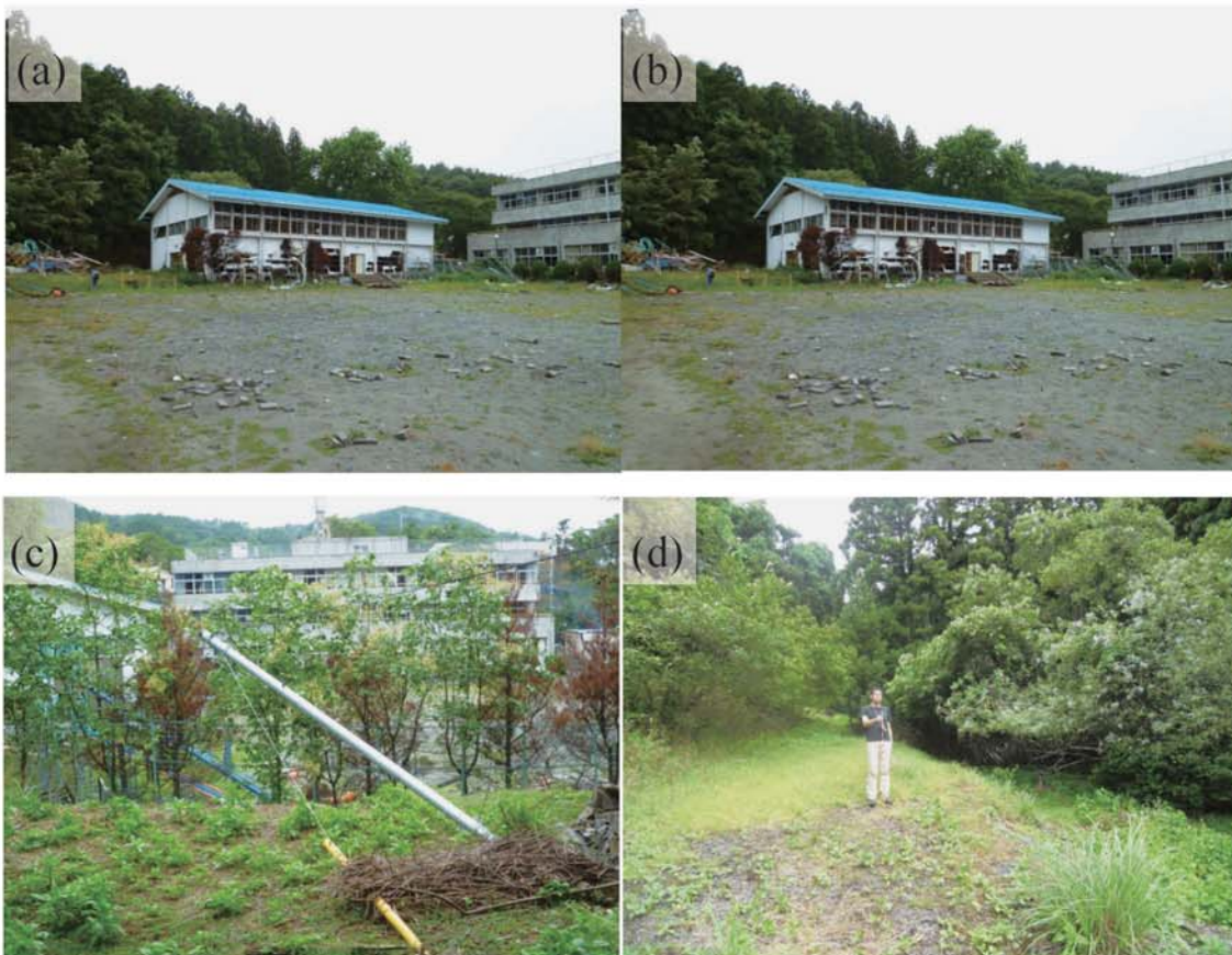
Fig. A216. (a)-(c) Damage at Oishiharahama. (d) Tsunami trace survey point at a slope behind the sixth Onagawa elementary school and the fourth junior high school (M62).
