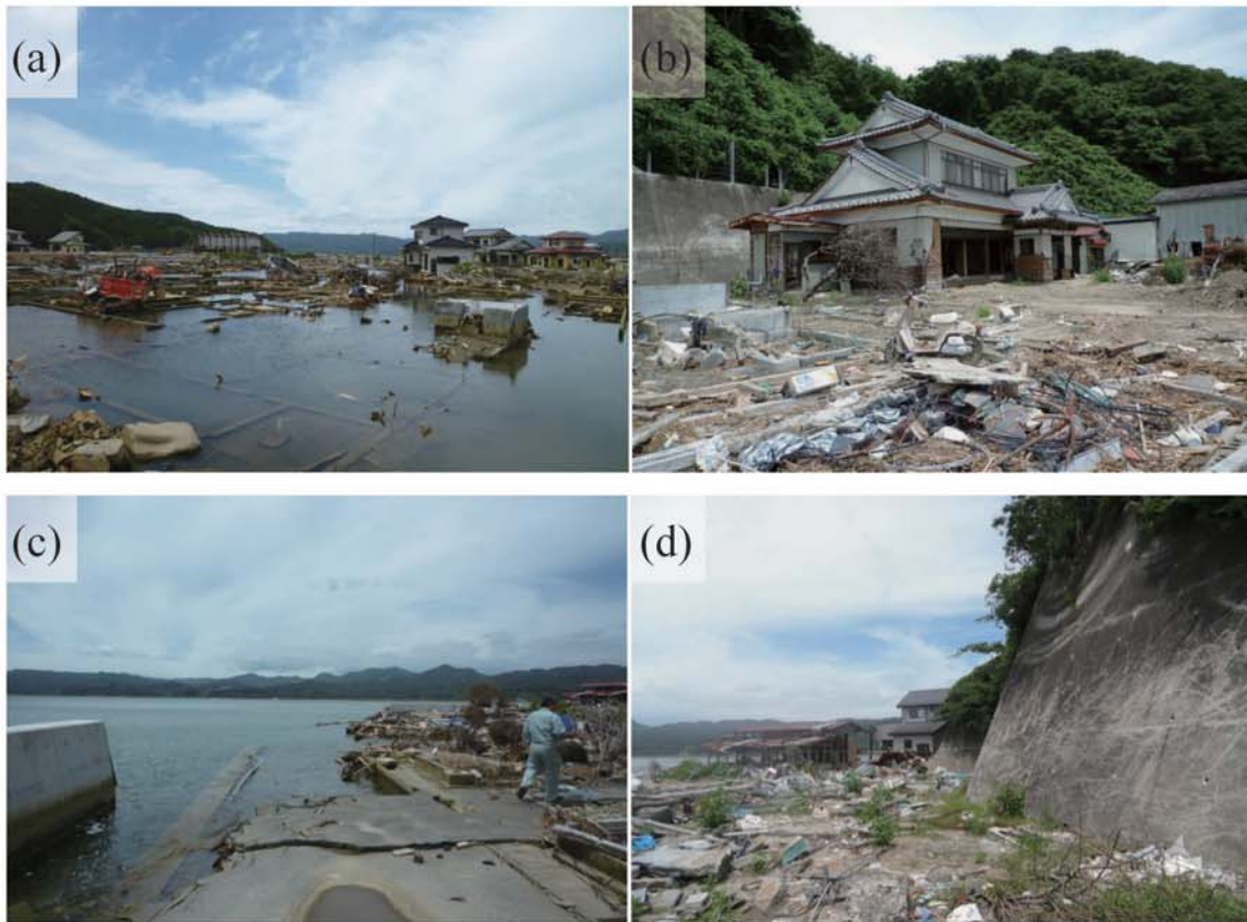
Fig. A190. (a)-(f) Damage at Onosaki and Nagatsura. (g) Tsunami trace survey point on a wall of Mr. Hamahata's house (2.46 m above floor level, M43). (h) Tsunami trace survey point on a wall of a house at a bridge in western Onosaki (0.32 m above second floor level, M44). (i) Tsunami trace survey point on a wall of a house facing northwest to the bridge at Onosaki (2.98 m above ground level, M45). (j) Tsunami trace survey point on a wall of a house on the eastern coast of Nakatsuraura (2.60 m above ground level, M46). (k) Tsunami trace survey point on a wall of Ryukokuji Kannondo (5.00 m above ground level, M47). (l) Tsunami trace survey point on a wall of Mr. Suzuki's house (5.57 m above ground level, M48).
