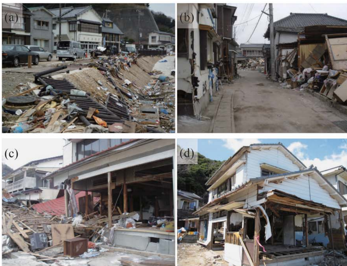
Fig. A240. (a)-(d) Damage at Hirakatacho. (e) Watermark on windowpanes of a house near Hirakata Fishing Port (1.95 m above ground level, B1). (f) Watermark on a window frame of the house at the right side of the figure (1.435 m above ground level, B2). (g) Watermark on windowpanes of entrance doors of Minshuku Yanagiya (0.89 m above ground level, B3). (h) Tsunami inundation limit at a slope behind a grave site (B4). (i) Tsunami inundated on the first step of a concrete stairway in a southern coastal residential area (B5).
