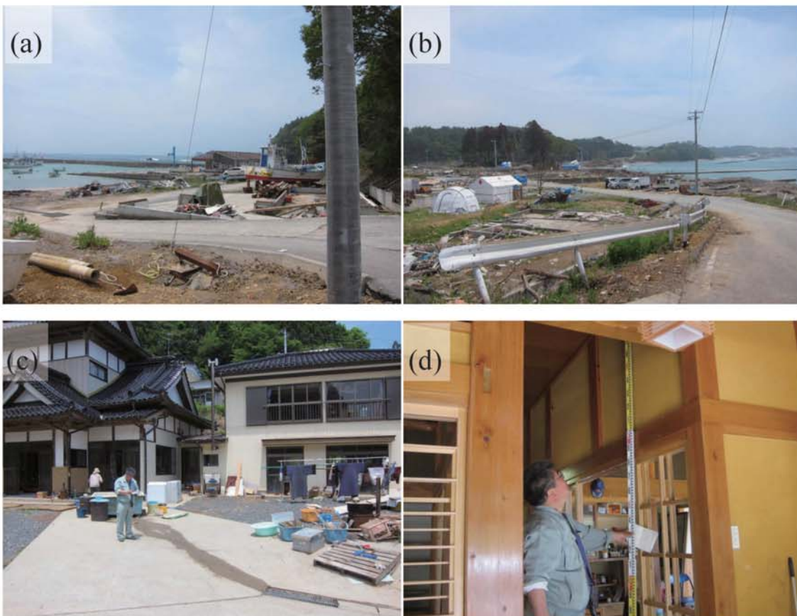
Fig. A164. (a)-(c) Damage at Utatsu-Tatehama. (d) Tsunami trace survey point on a wall of Mr. Chiba's house (3.04 m above the dirt floor, M27).
