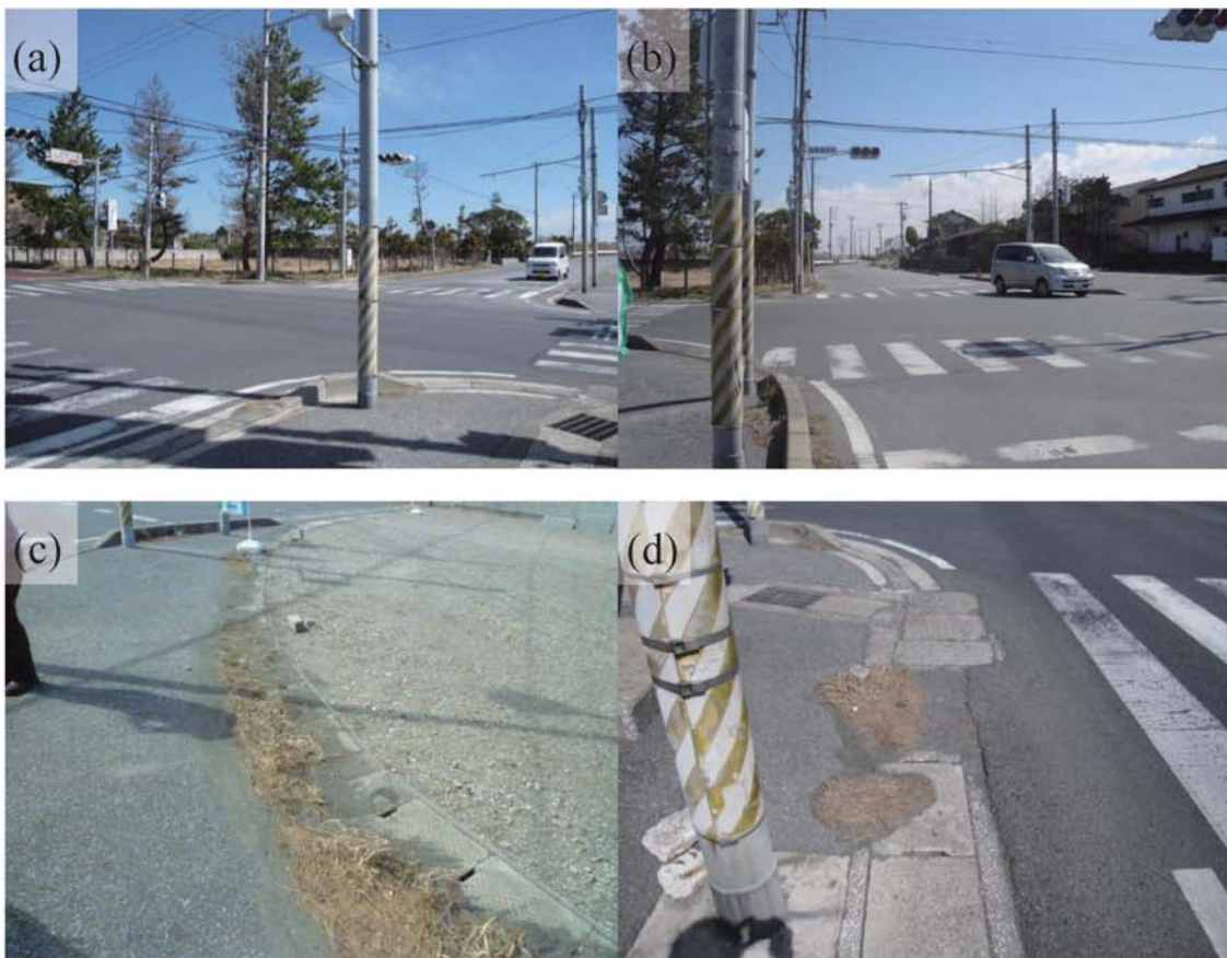
Fig. A320. (a)-(b) Crossroads inundated by the tsunami at Ichinomiya. (c)-(d) Tsunami trace survey point at a drift close to the crossroads (C19).
