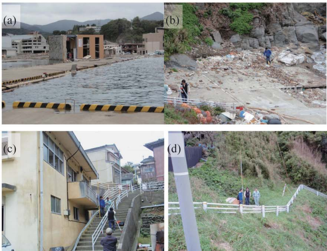
Fig. A218. (a)-(b) Damage at Enoshima. (c) Tsunami trace survey point on a wall of the fishermen's cooperative building (M63). (d) Tsunami trace survey point near a well (M64).
