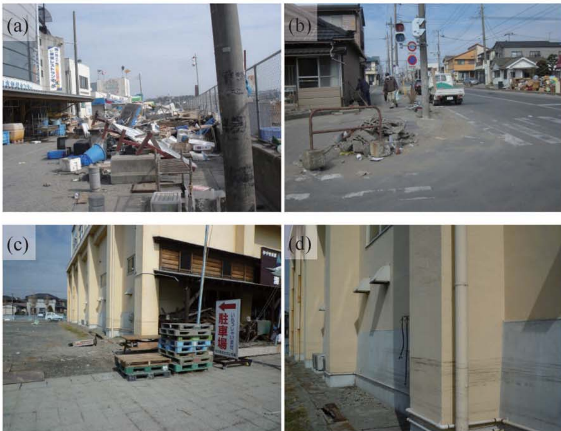
Fig. A282. (a)-(b) Damage at Kaimoncho (Nakaminato Fishing Port). (c) Building of fish market in the port (tsunami trace survey point). (d) Watermark on a wall of the market building (1.19 m above ground level, B29).
