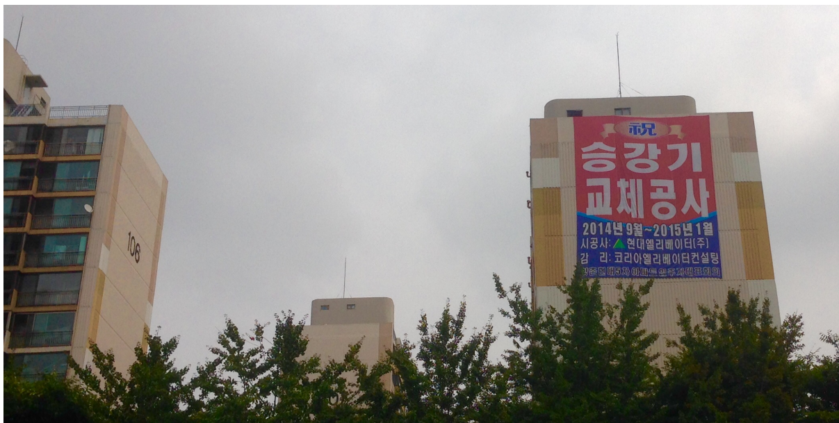
Figure 8-2. PR banner for notifying the replacement elevator by resident committee
