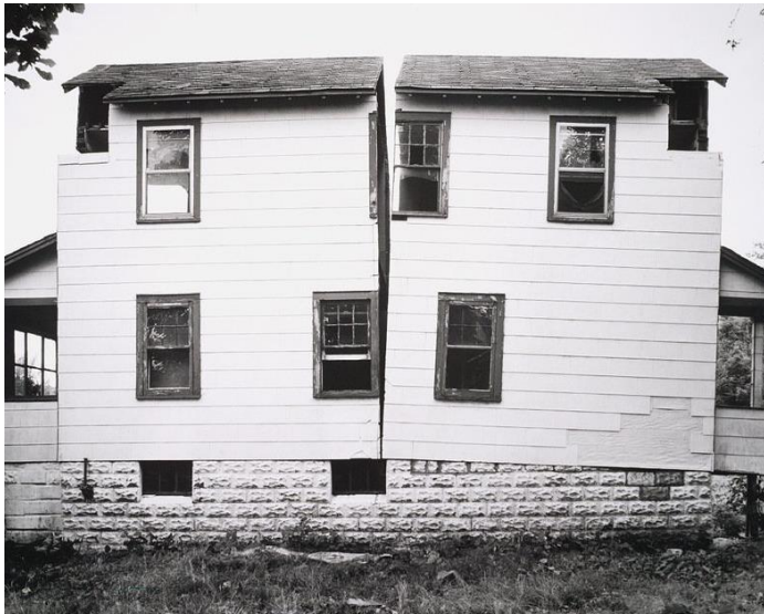
Gordon Matta-Clark, Building cuts , década de 70.
