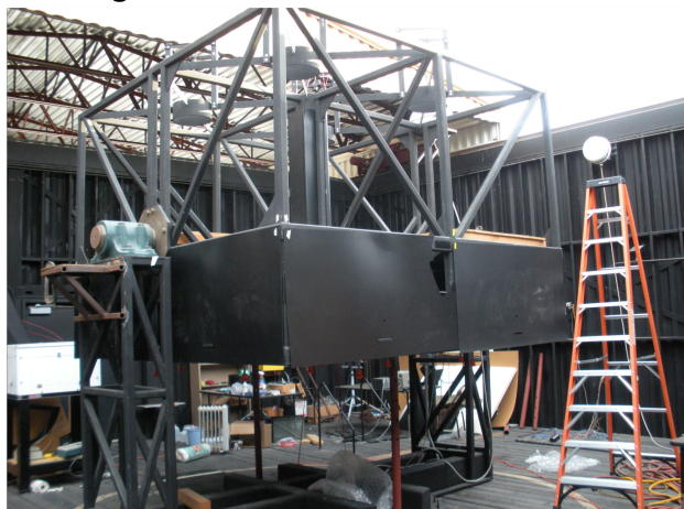
The cage structure which holds the 4 mirrors
