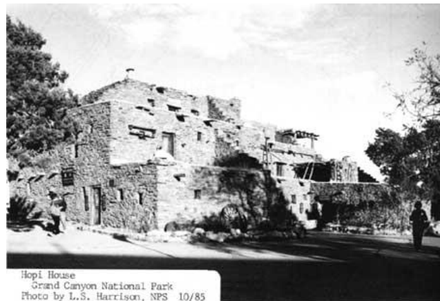
Figure 1.3: Hopi House: The Hopi House is constructed of stone masonry and embellished with mud plaster. Photo courtesy: www.nps.gov
