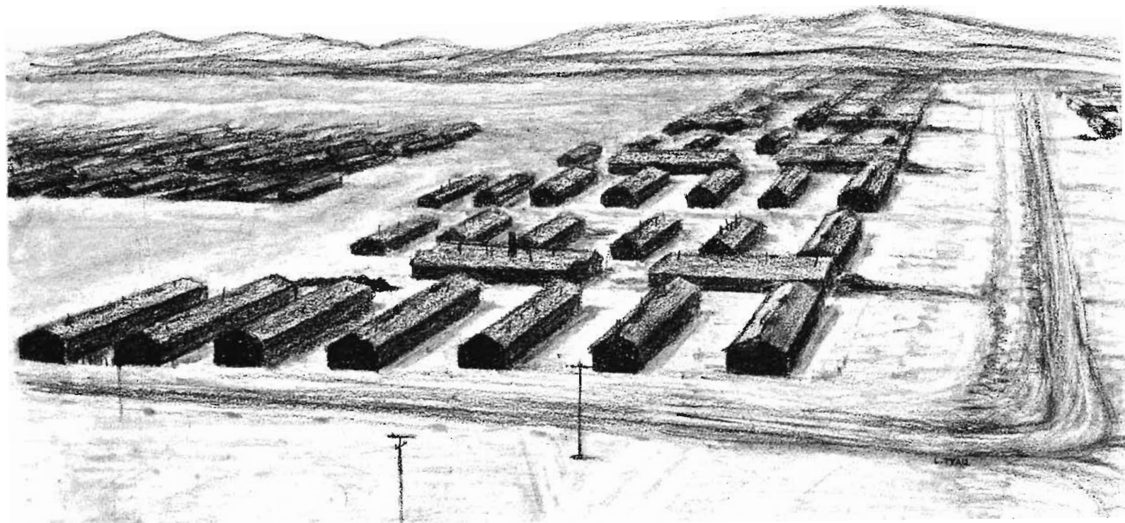
CENTRAL UTAH RELOCATION CENTER Millard County, Utah, 1942-1945
