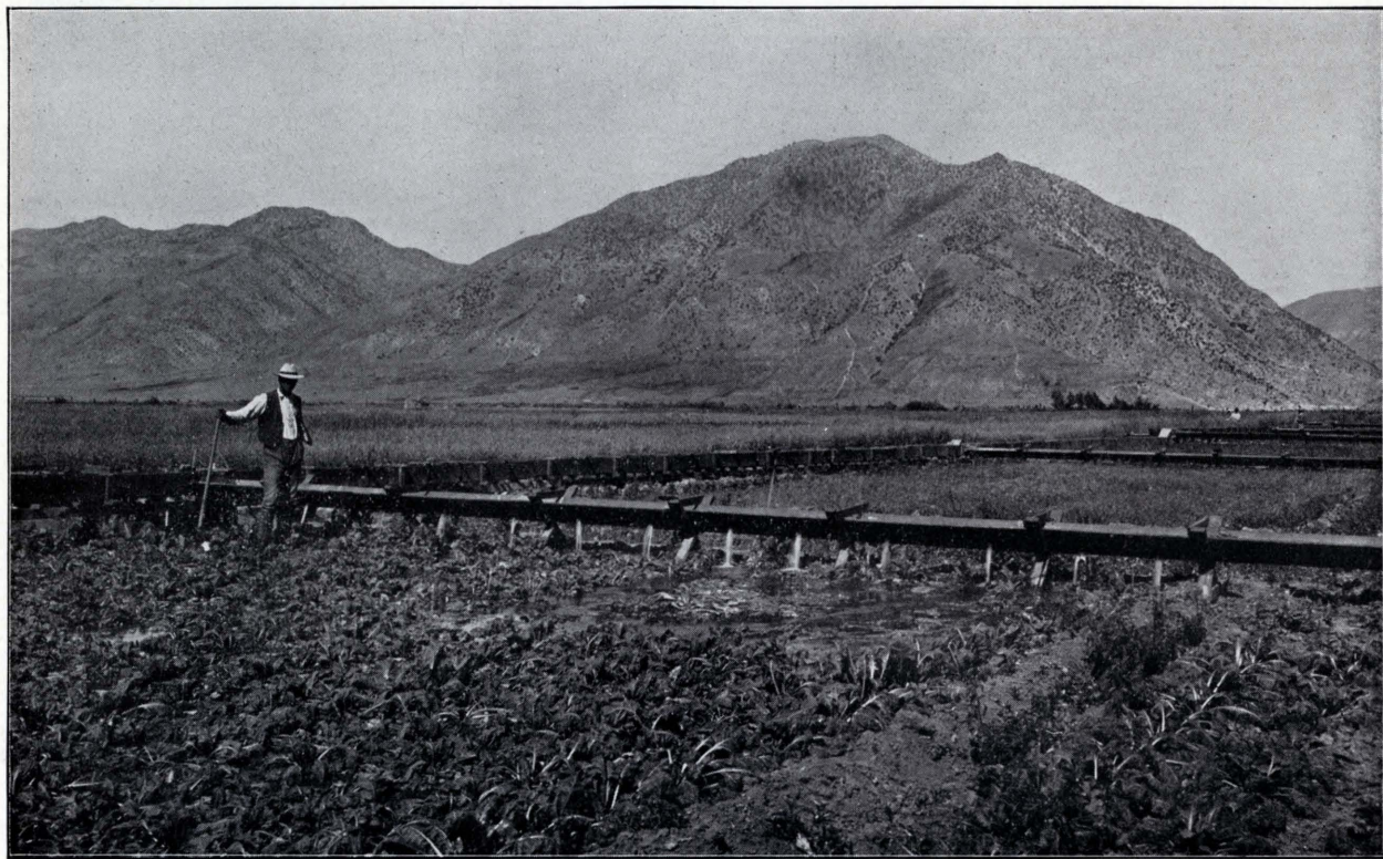
Plate 8. Method of applying measured quantities to the experimental plats.
