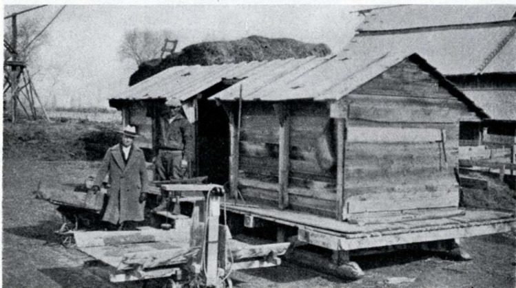
Figure 1—Movable granary and hay scales used for weighing grain and hay in lamb-feeding experiments at Monroe.
