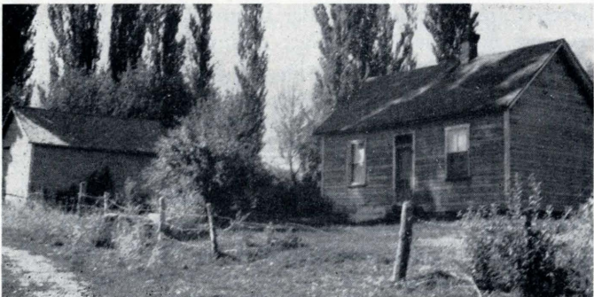
A village farm home in poor condition
