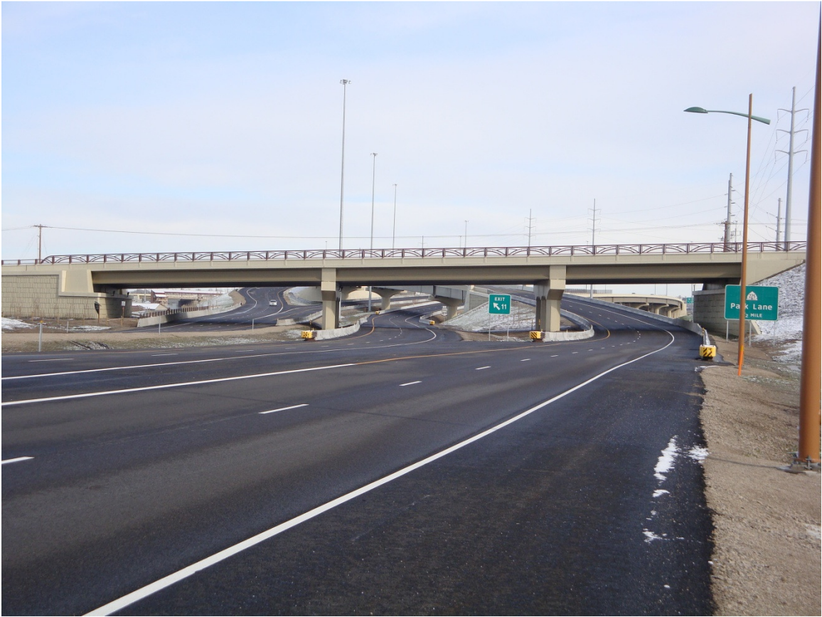
Figure 4.4 669 Bridge looking north.
