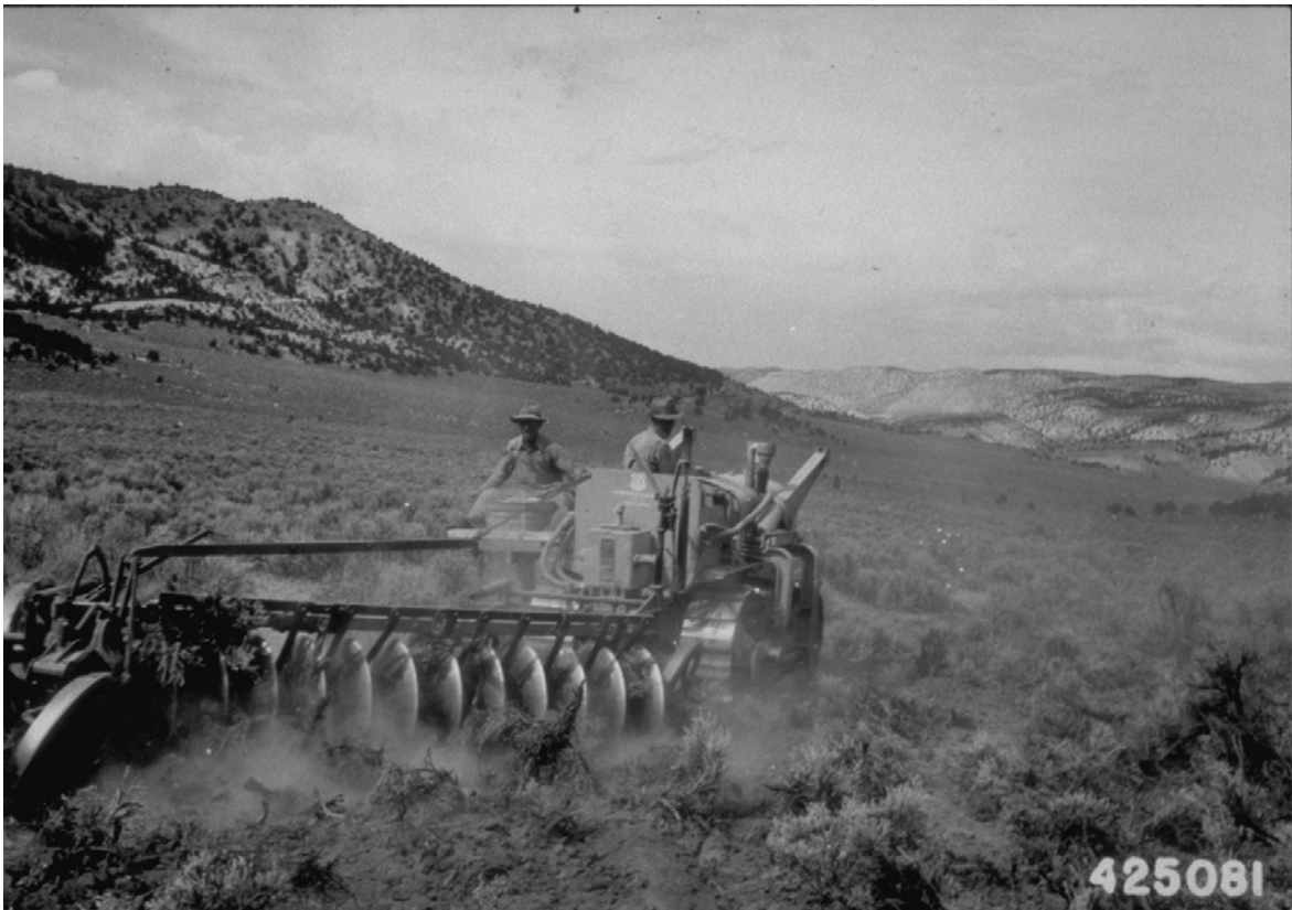
Figure 11. Charles Demoisy, Tractor-Drawn Wheatland Type Disc Harrow Clearing Sage and Preparing Seedbed for Grasses, The Rocks, Soldier Fork, Fish Lake National Forest, 4 September 1942 , Courtesy of FS Region 4 Ogden, Utah.
