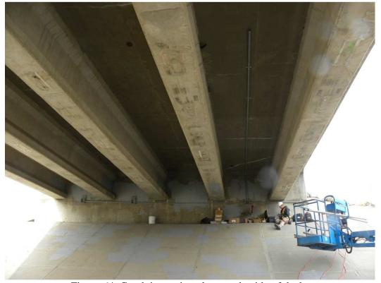
Figure 64. Conduit running along underside of deck.
