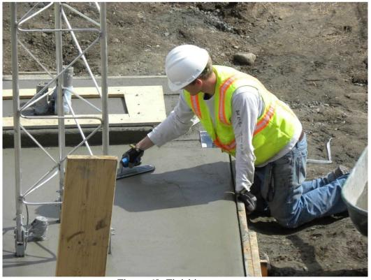
Figure 60. Finishing concrete.
