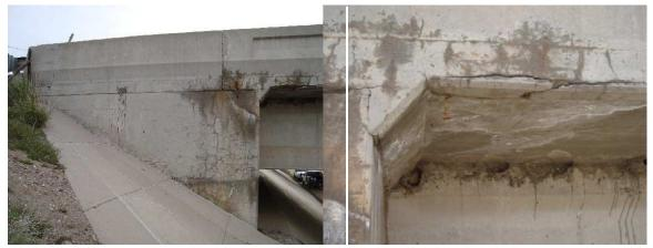
Figure 4. Cracking at abutment.
