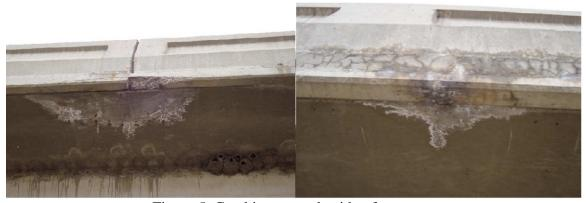
Figure 5. Cracking on underside of parapet.
