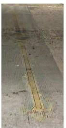
Figure 23: Quartz based WIM as seen installed in a lane leading to Perry, Utah Port of Entry.
