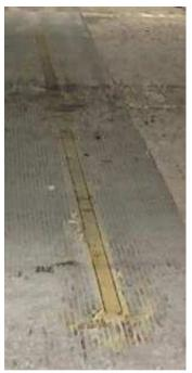
Figure 52. Quartz based WIM installed in lane leading to Perry, Utah Port of Entry.
