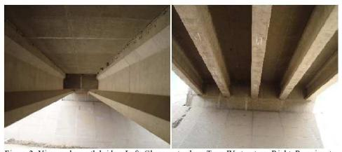
Figure 2: View underneath bridge. Left: Close-up to show Type IV structure. Right: Pan view to show all five girders.
