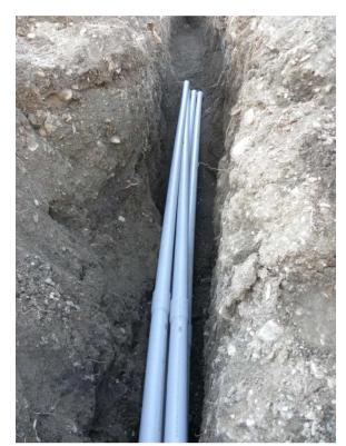
Figure 58. Conduit running from pad to bridge.
