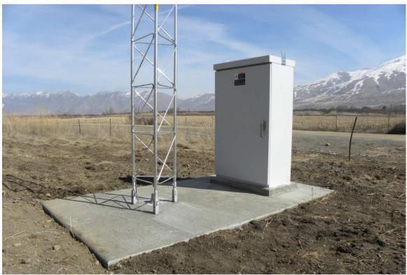
Figure 61. Insturment pad with installed tower and cabinet after grading.
