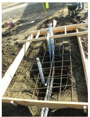
Figure 57. Pad form and reinforcing steel.
