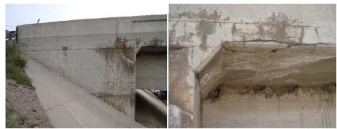
Figure 3: Cracking at Abutment.
