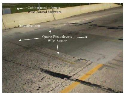
Figure 24: WIM installed on lane leading to Perry, Utah Weigh Station. See labeling for part descriptions
