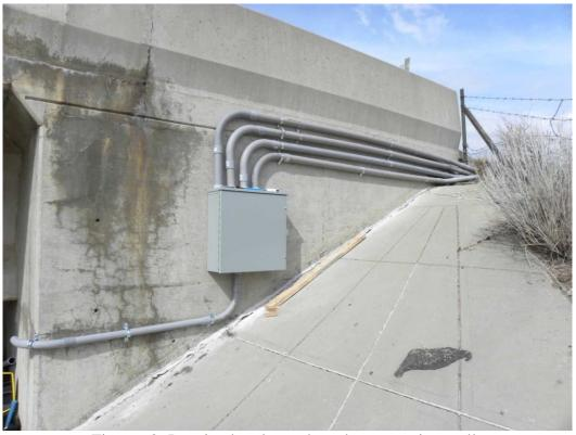
Figure 62. Junction box loacted on abutment wing-wall.
