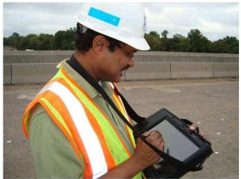
Figure 4: Recording distress data in an electronic notebook.
