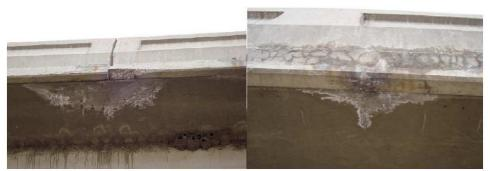
Figure 4: Cracking on underside of parapet.
