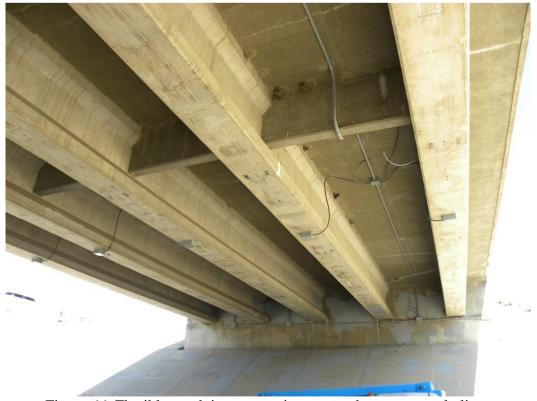
Figure 66. Flexible conduit connects instrument boxes to supply line.
