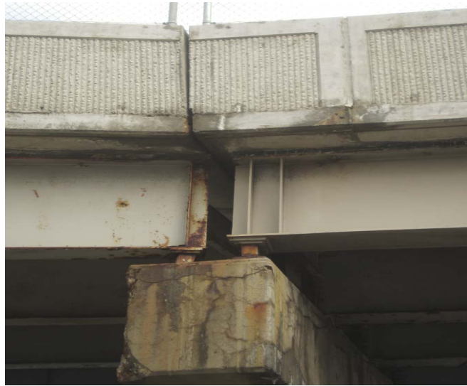
Fig 3.37 Supports at the pier caps.
