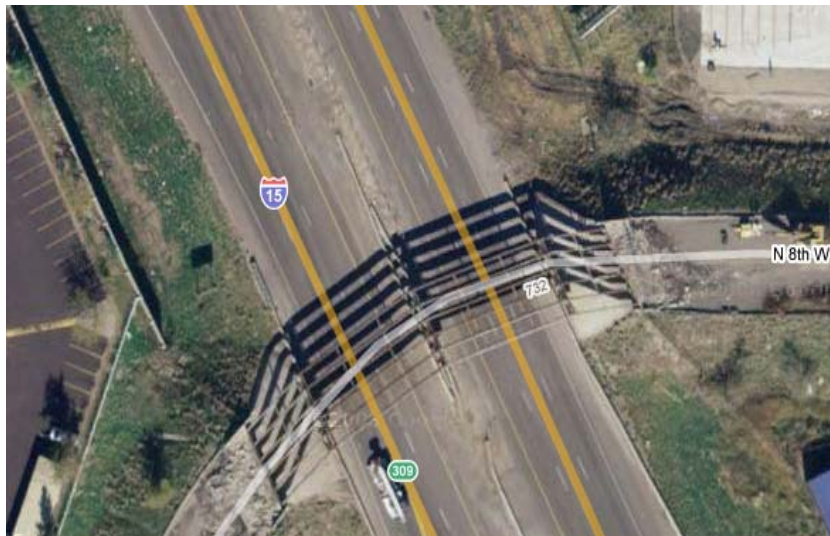
Fig 3.1 Aerial view of the 8 th North Bridge.
