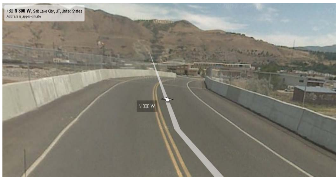
Fig 3.8 Barriers and concrete deck on the 8 th North Bridge.
