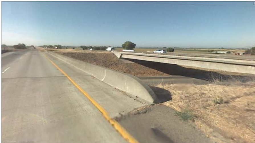
Fig 4.5 View of the barriers on the bridge.
