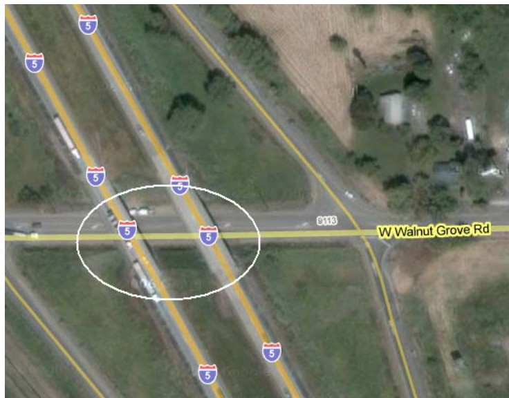
Fig 4.1 Aerial view of the Walnut Grove Road Bridge.
