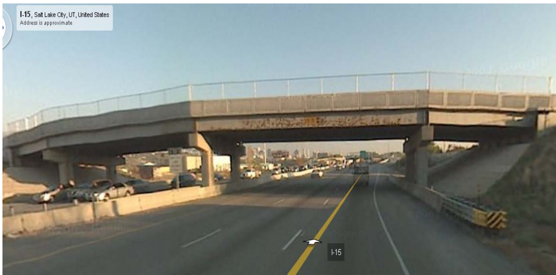
Fig 3.2 8 th North Bridge view from I-15 Freeway.
