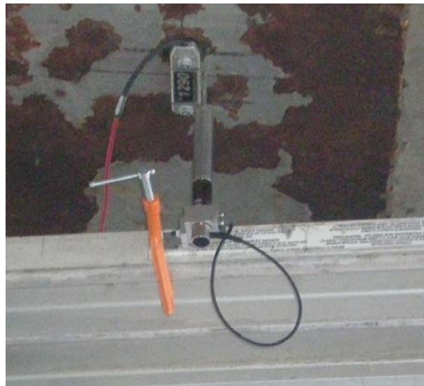
Fig 3.18 Typical LVDT sensor used in the live load test.
