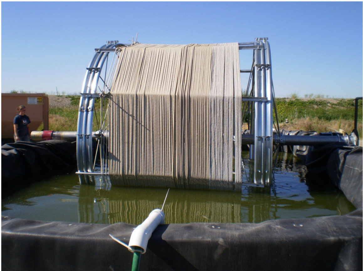
Figure 2: A Pilot Scale RABR Unit. (Logan, UT Municipal Wastewater Treatment Plant)
