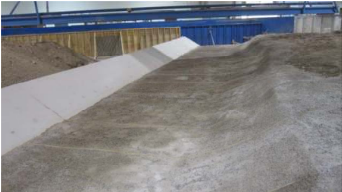
Figure A3. Upstream view of the canal with topography (Rahmeyer et al. 2010).
