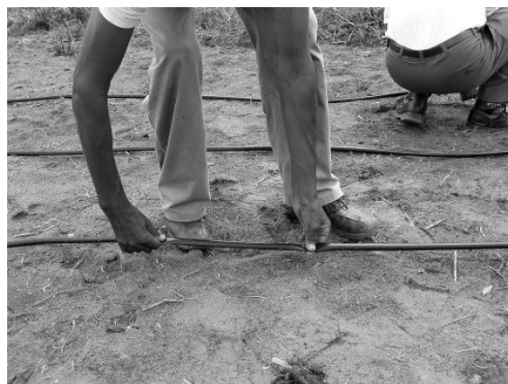
Fig. H.30. Stretching the lateral cross-section by increasing the pressure
