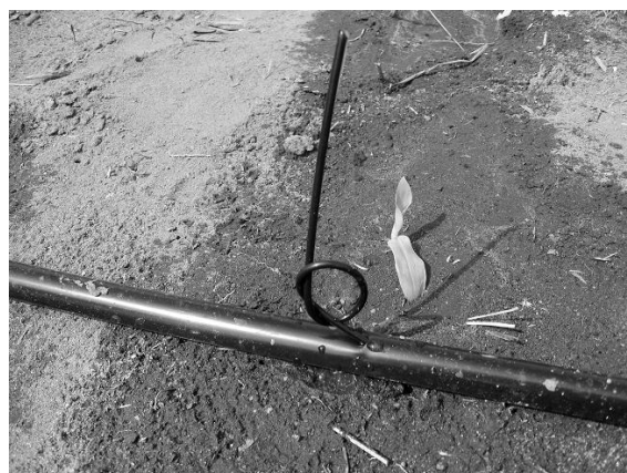
Fig. H.36. Emitter inserted to less than 1 cm. EC2.
