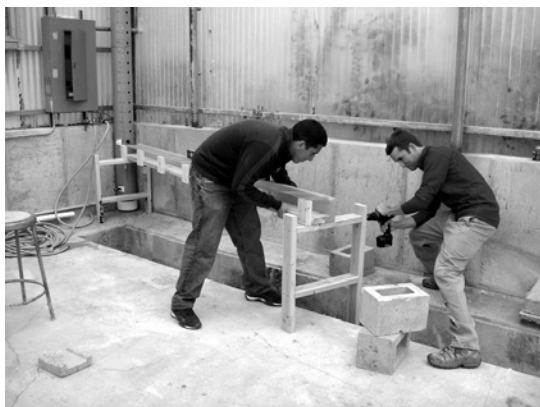
Fig. B.1. Runway construction. The lateral was constructed in 3-m sections.
