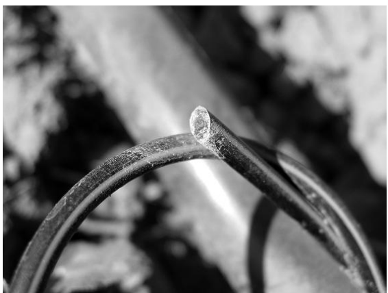
Fig. H.29. Emitter outlet clogged from discharging into soil. AGFTC.
