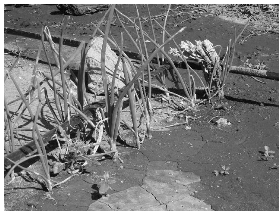
Fig. H.18. Lateral and submain tension. This caused the lateral to be elevated above ground. FTC2.
