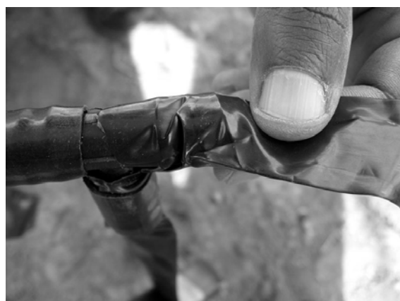
Fig. H.40. Lateral folded at submain tee. Golba1.
