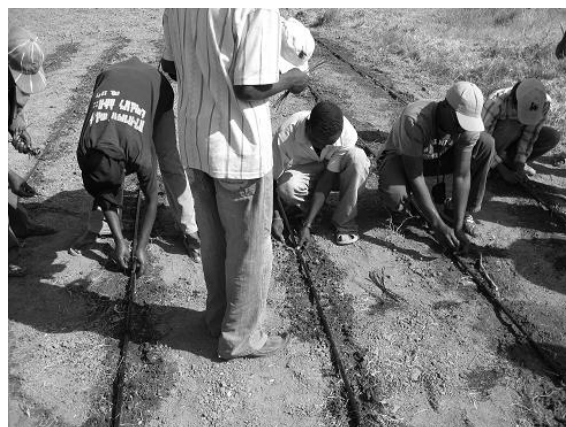
Fig. H.32. Punching holes in the lateral for emitter insertion
