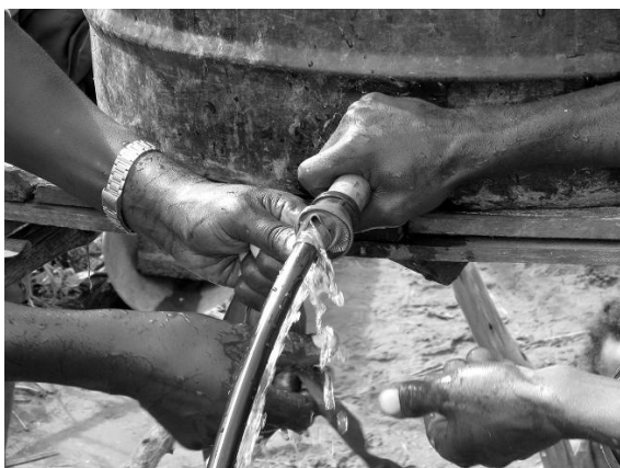
Fig. H.33. Mainline inserted directly into the header tank outlet spout. EC2.
