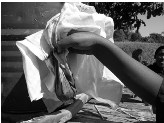
Fig. H.43. Debris filtered from the water before entering the header tank. ANFTC.
