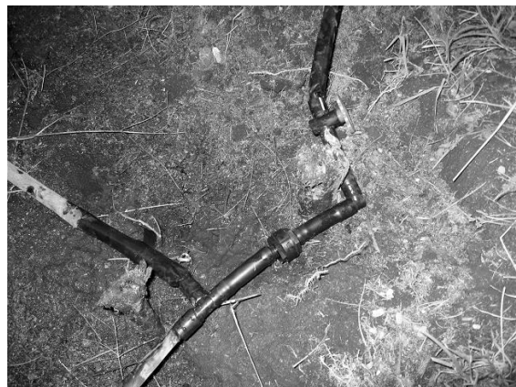
Fig. H.20. Improper placement of the header bag. This causes kinks in the laterals and mainline DH1.
