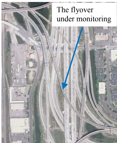
Figure 7. The aerial view of the bridge under monitoring
