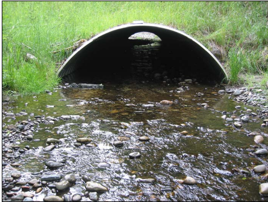
Figure 1. Example of a buried-invert culvert.
