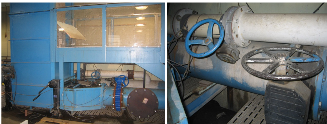
Fig. 3-6. Supply piping to the rectangular flume test facility
