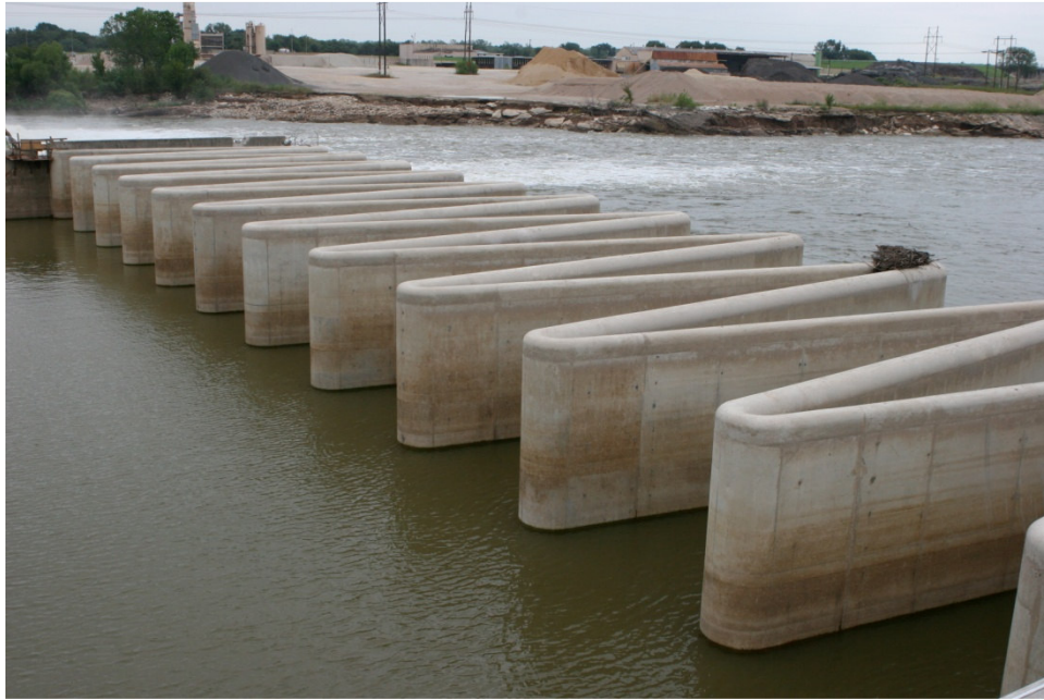
Fig. 2-4. Rounded apices of Brazos Dam, Texas, USA
