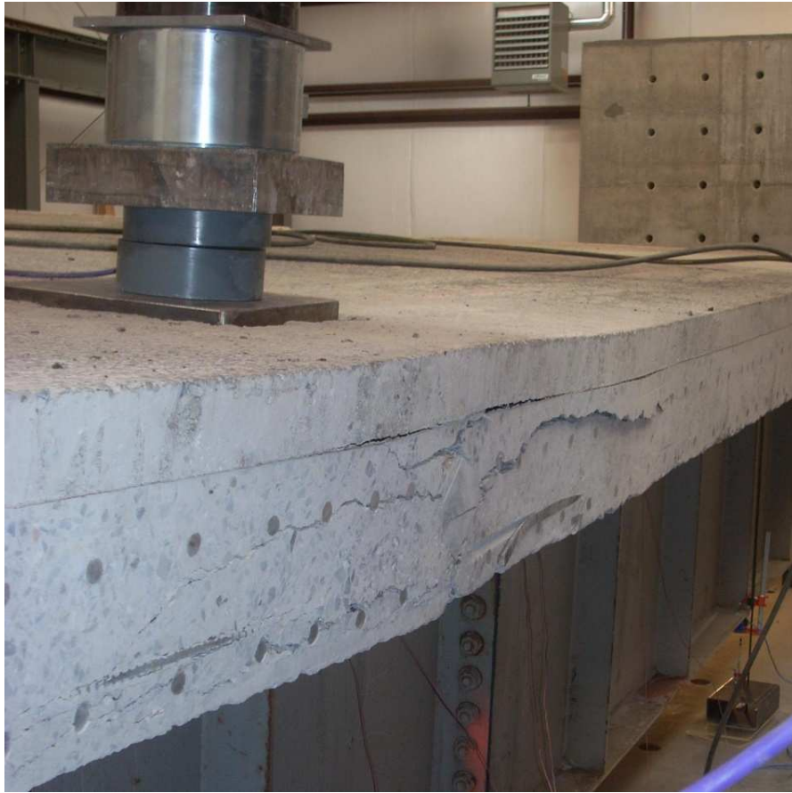
Figure 15. Splitting failure in concrete deck.
