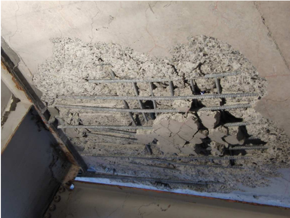
Figure 26. Underside of deck after Punching Shear Test 2 failure.
