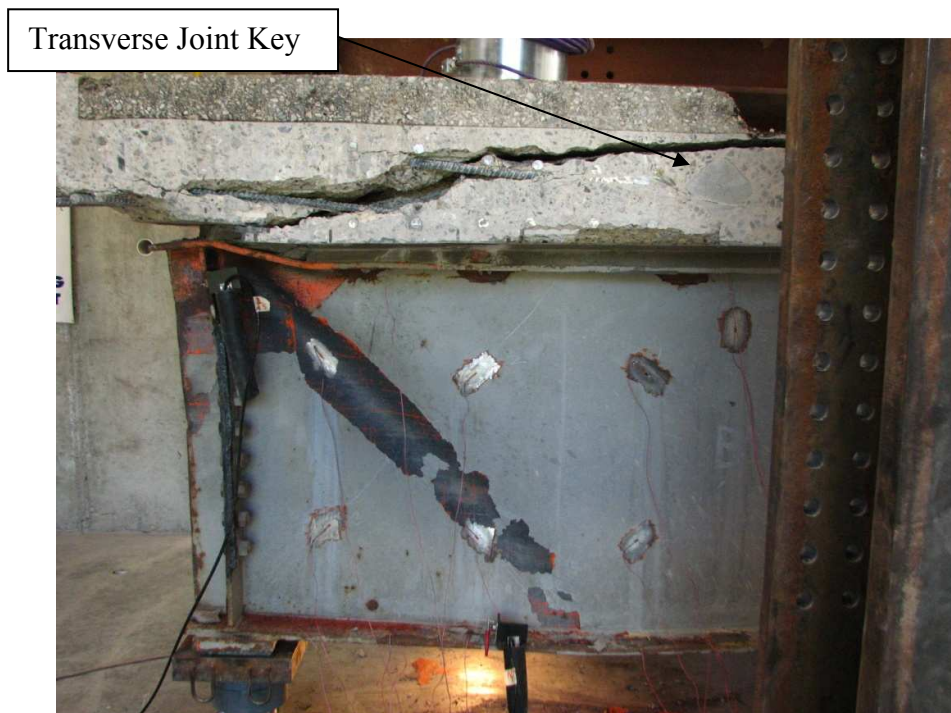
Figure 21. Beam Shear Test B failure.
