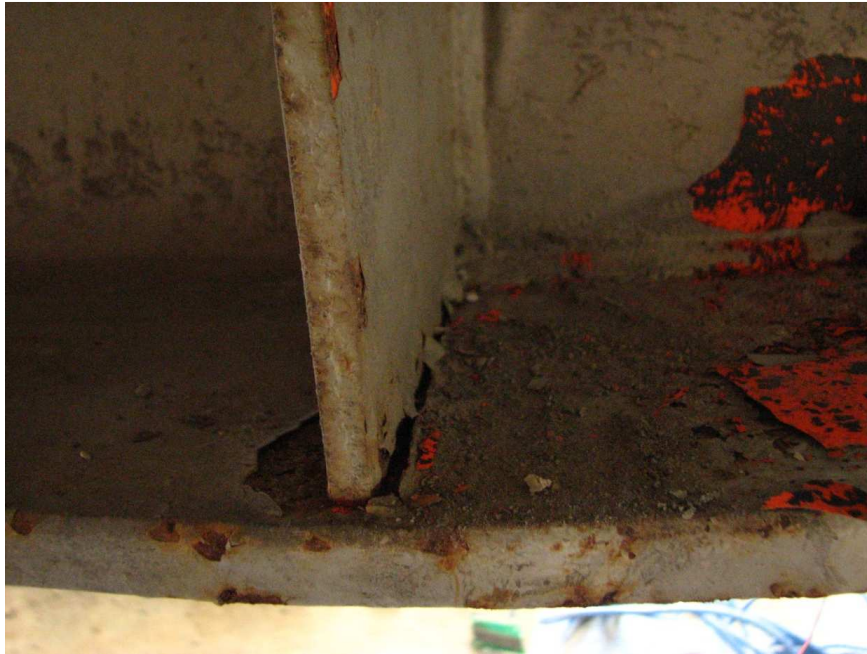
Figure 24. Web stiffener displacement after Beam Shear Test B.
