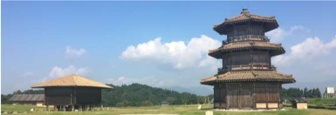
Figure 6.18 The Restoration at the Kikuchi Castle (Source: Photos by the author)
