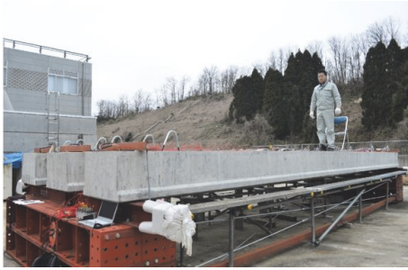
FIGURE 5: Impact test and sensor layout on the PC girder.
