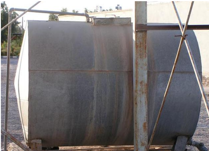
Photo 3.36- Water Tank 1, Aflatoonian Hospital
