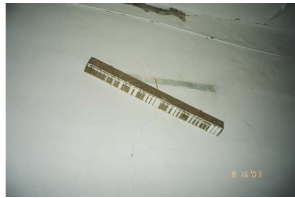
Photo 3.14- Damage to electric equipment CHU Hospital
