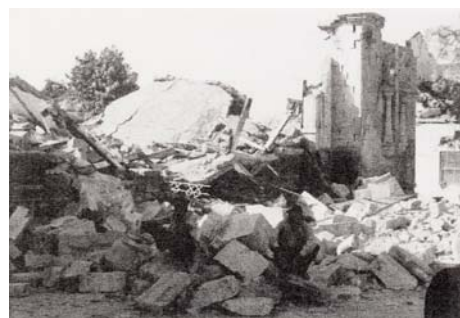
Photo 3.10- Collapsed Jubilee Hospital
