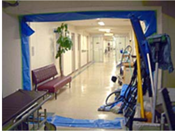
Photo 3.53- Damage to separation joint
