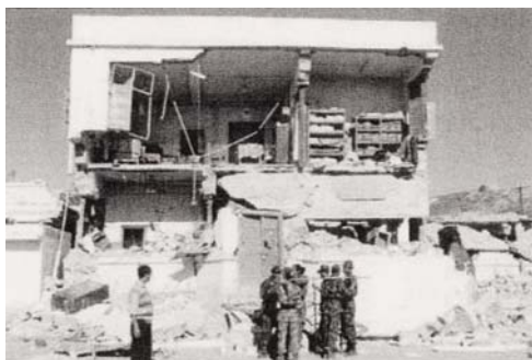
Photo 3.9- Collapsed Bhuj Central Hospital
