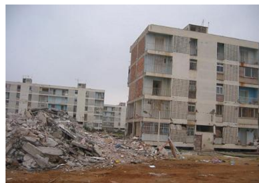
Photo 3.12- Collapse of residential building
