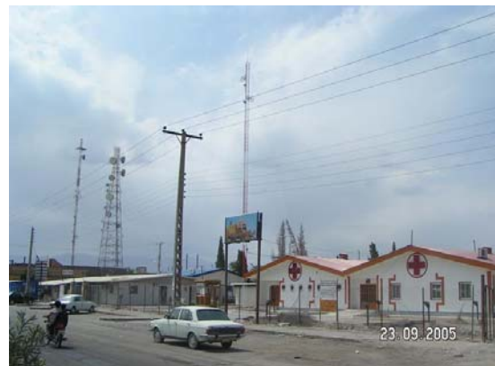
Photo 3.48- Prefabricated buildings installed instead of the Imam Khomeini Hospital September 2005
