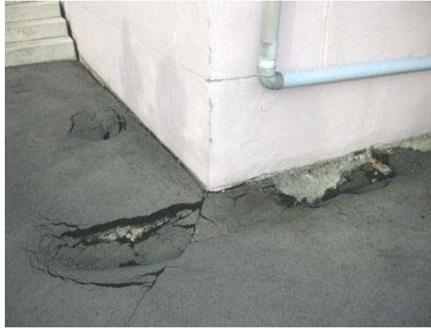
Photo 3.57- Liquefied soil
