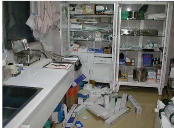
Photo 4.8- Equipment toppled from selves
