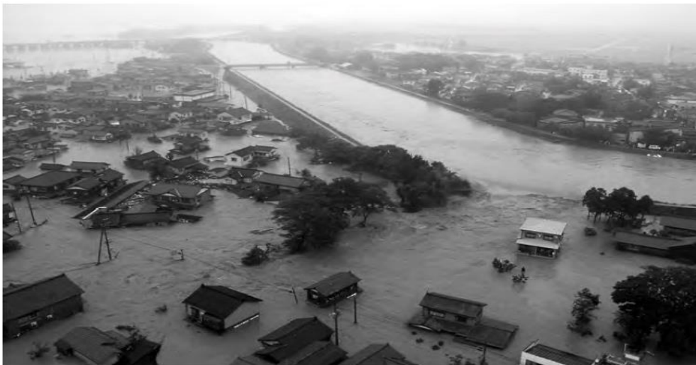
Figure 9: Flood water flowing into the housing area from the bank of the Kariyata River (NIED, 2006)
