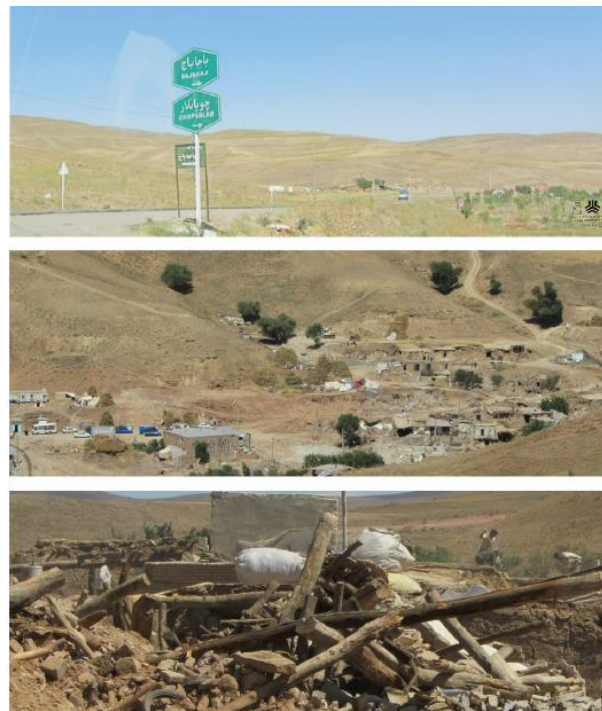
Fig.4.14 Field observation of Chopanlar showing the collapsed buildings.
