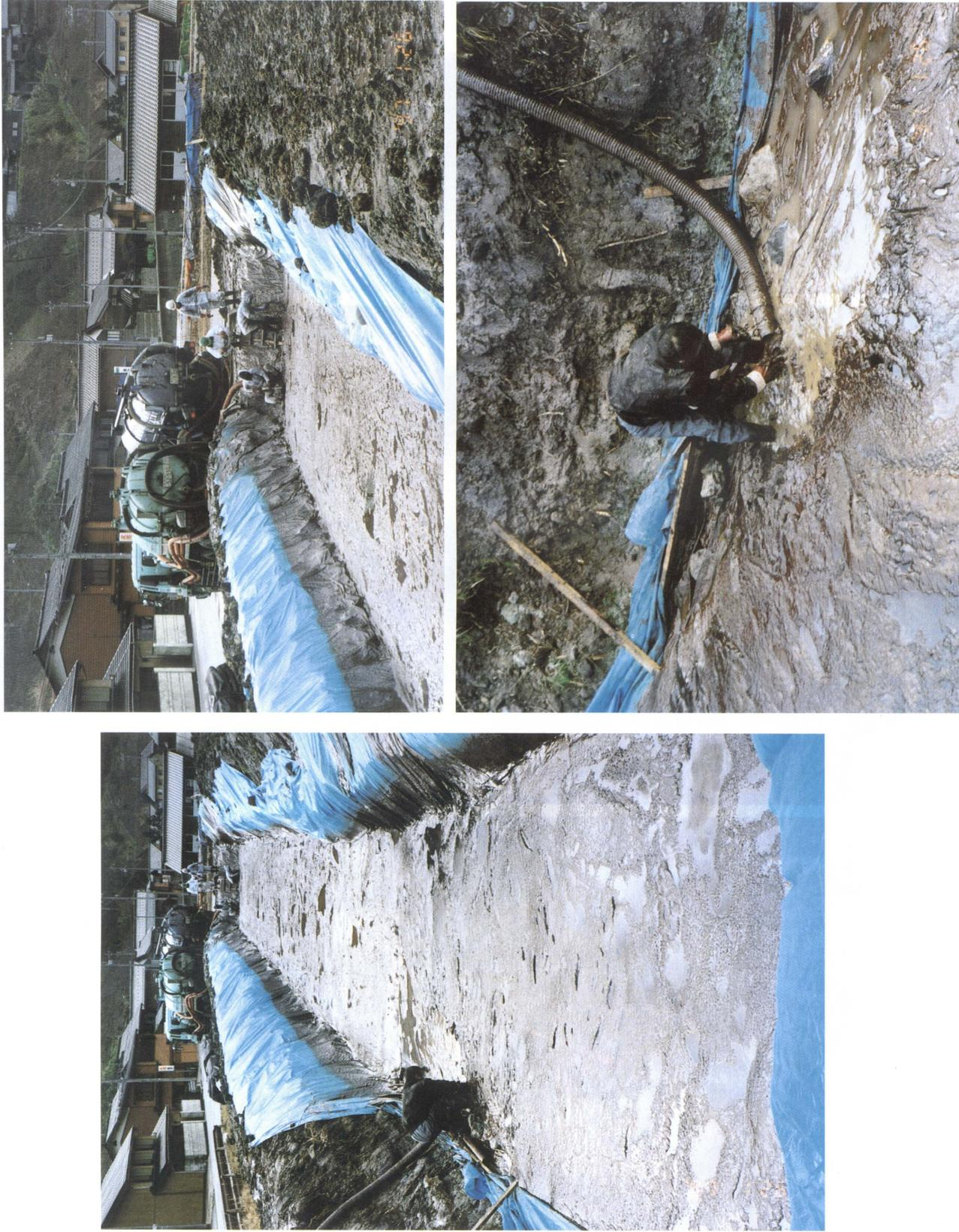
**Figure 14** Quick – made pool covered with plastic sheet in rice field to keep heavy oil collected from Sosogi seashore in Wajima City (left). Vacuum truck carrying the oil to waste plants (right upper), and the heavy oil was too viscous to suck, so a man was helping the machine (right down) (January 26<sup>th</sup>, 1997).
