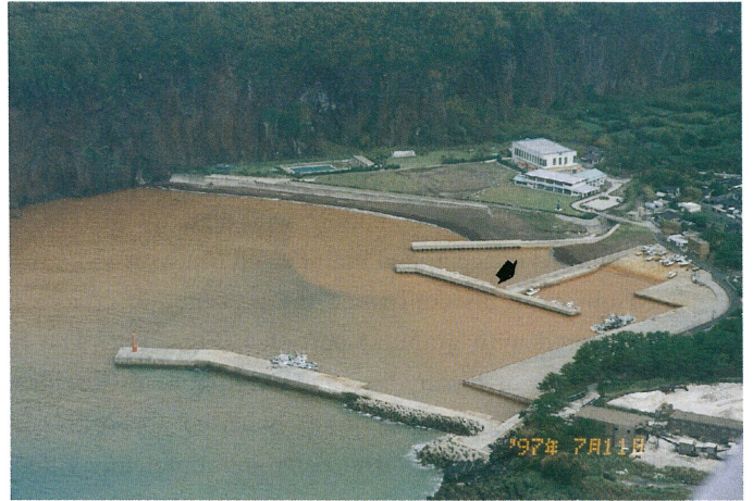
Fig. 1 An overall view of the breakwaters at Nagahama Port. The arrow shows the location of the terrace-like sediments .
