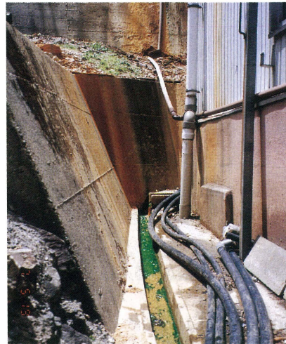
Fig. 1 Solidified reddish brown biomats on the walls around spring pipes and soft reddish brown biomats 1~2 cm in thickness and green biomats occur along drainage ways.
