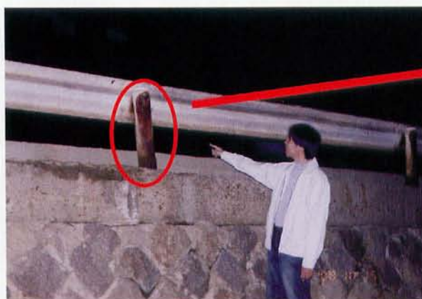
Fig. 5. The metallic guardrail has rusted (circled) after volunteers attempted to soak up crude oil on Mallipo Beach using a high-temperature and high-pressure nozzle. Images are for before washing (January) and after washing (October 2008).
