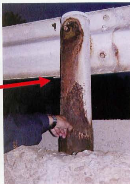
Fig. 5. The metallic guardrail has rusted (circled) after volunteers attempted to soak up crude oil on Mallipo Beach using a high-temperature and high-pressure nozzle. Images are for before washing (January) and after washing (October 2008).
