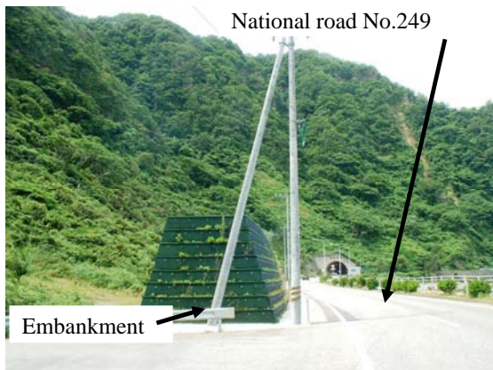
Fig. 14. Constructed embankment against rockfalls.
