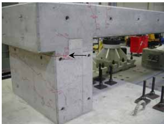
Photo 3. Opened crack at construction joint
