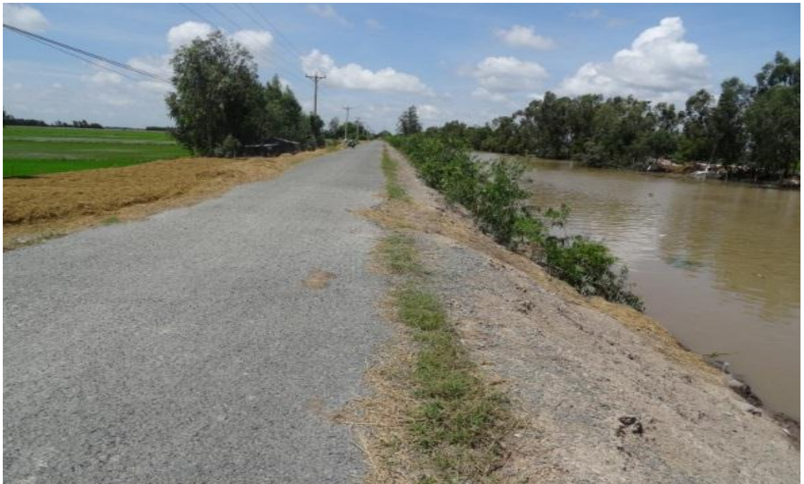
Figure 3.2: High dyke in An Giang (i.e., dyke is >3 metres high and 12 metres wide) Source: Author (2015)
