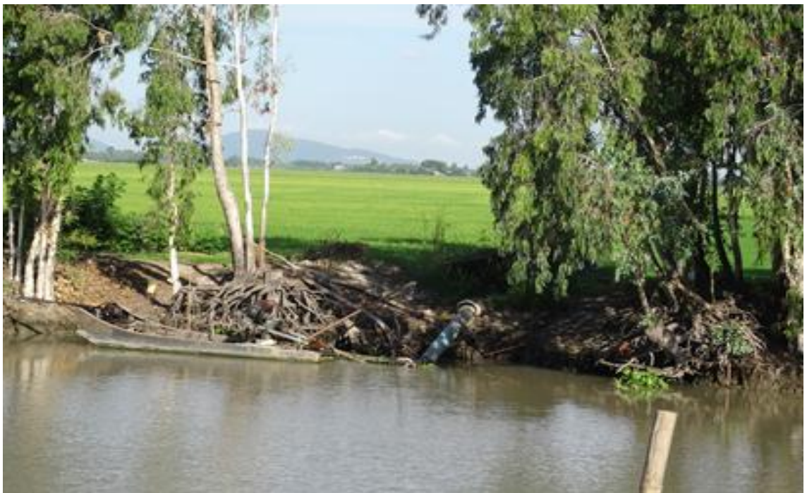
Figure 3.3: Low dyke in An Giang province (i.e., dyke is <2 metres high and 3 metres wide) Source: Author (2015)
