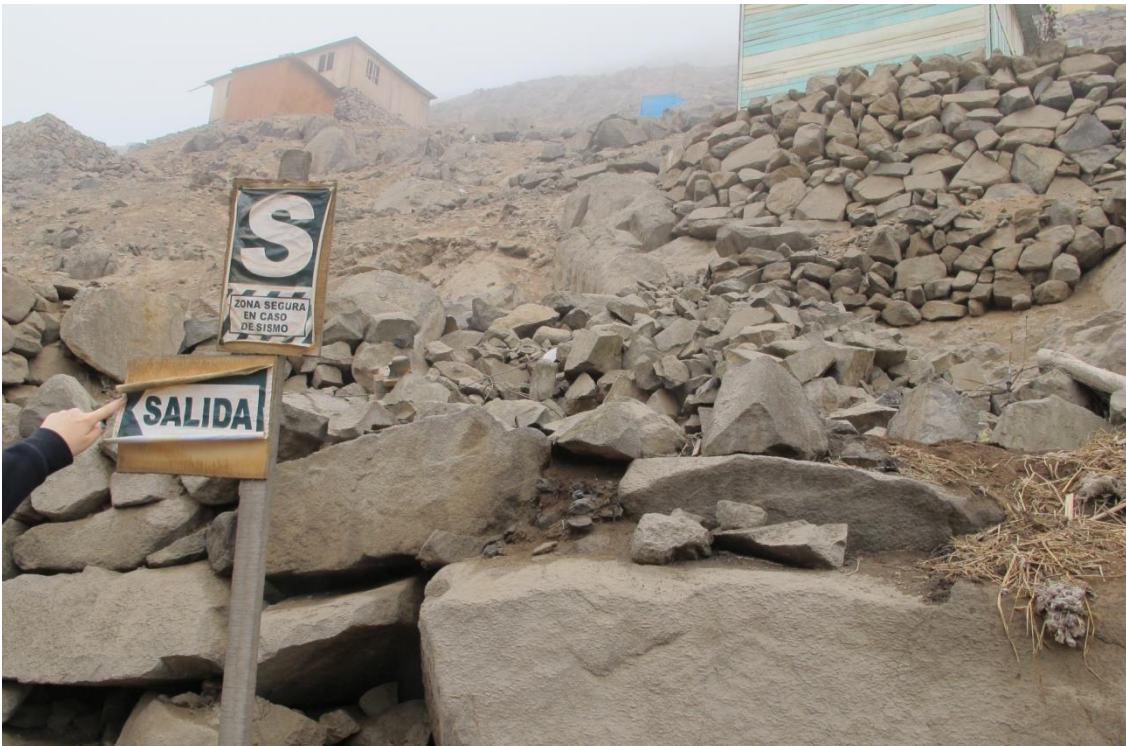
Figure 6.29: Evacuation route under potentially unstable retention walls and rocks.
