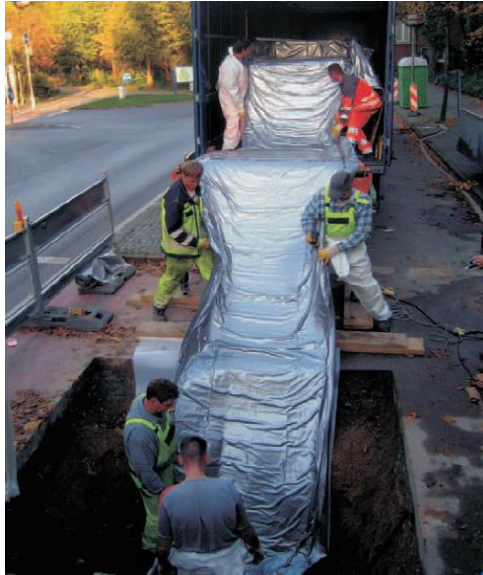
Fig. 2: Installation of CIPP in pipeline through pulled in place [Dilg 2007]
