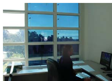
Fig. 3: SageGlass® EC windows in coloured and bleached state (with sensors inside the room monitoring the temperature and light transmission of the windows).
