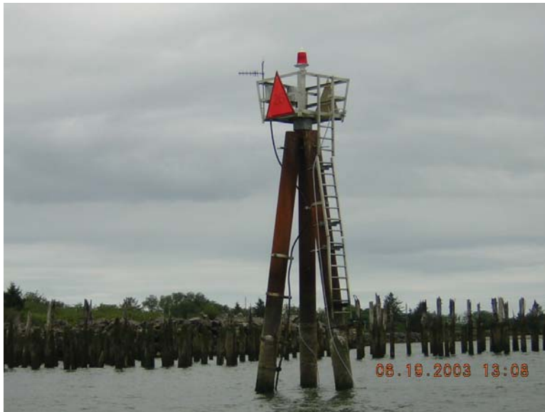
Figure 2-1: A Sensor Station of ALERT System [15]
