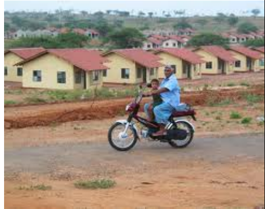
Figure 5.6: Tsunami housing Sources: UDA Archive
