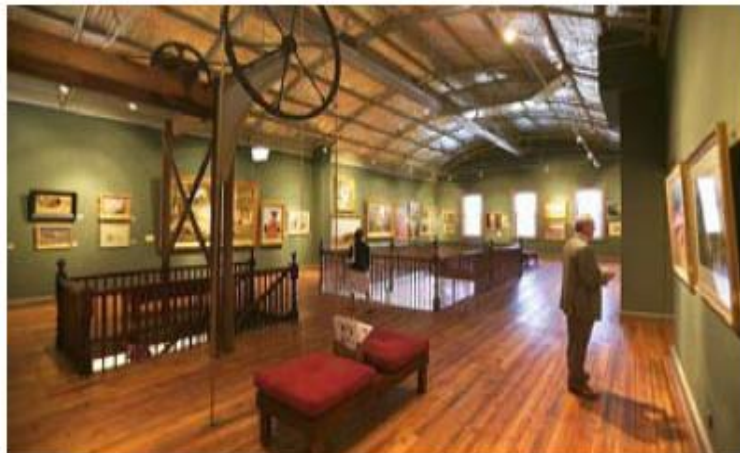
82 : The original curved roof has been lined, while still exposing the significant 1889 light metal truss.
