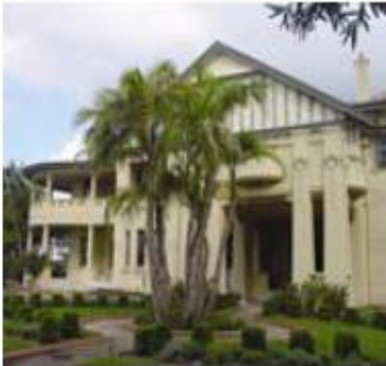
59 : Babworth House after its adaptation for apartments.
