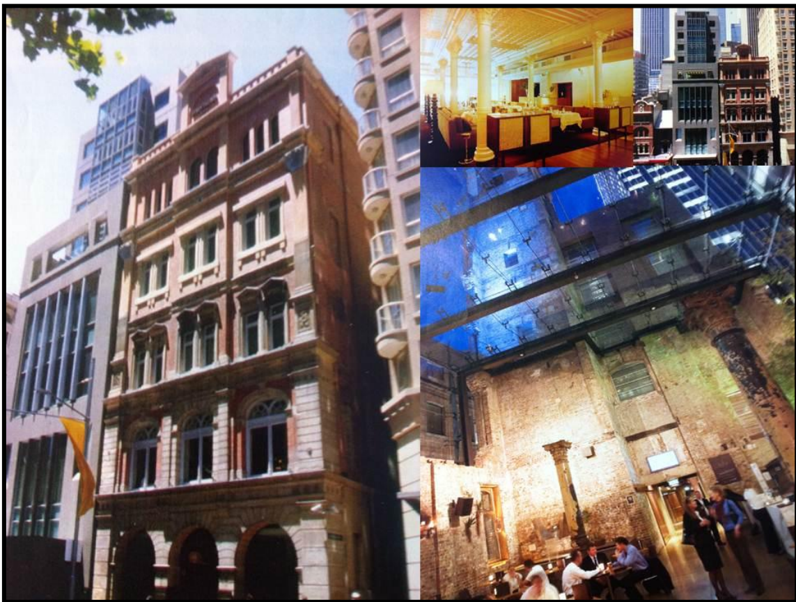
FIGURE 4-14 GEORGE PATTERSON WAREHOUSE
