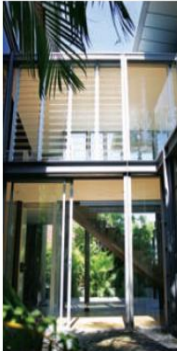
70 : The rear elevations allow maximum natural air movement.
