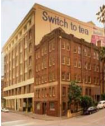
71 : The Bushells Building with its repainted façade and reinstated signage.
