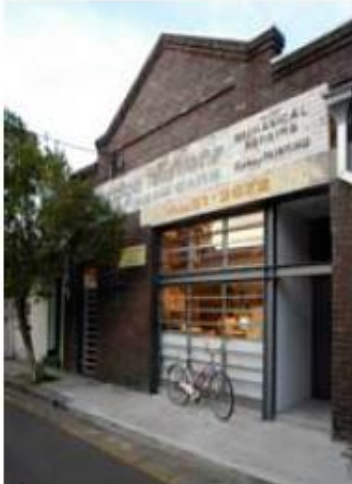
55 : Egan Street, Newtown has been adapted for apartments and a studio space for a collective of architects.
