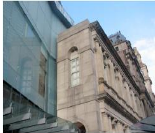
Figure 6. GPO MELBOURNE EXTERIOR (SHOWING NEW EXTENSION)
