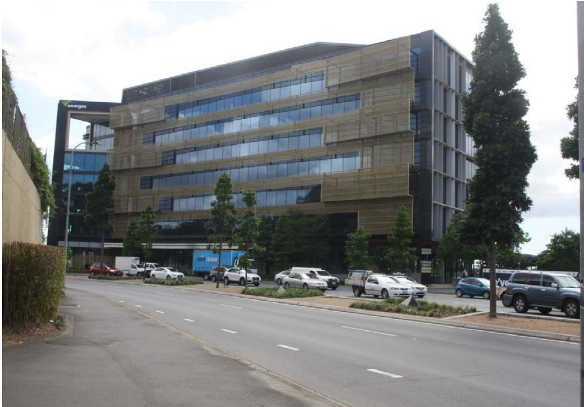
Figure 4.1 Energex Building, Newstead Riverpark
