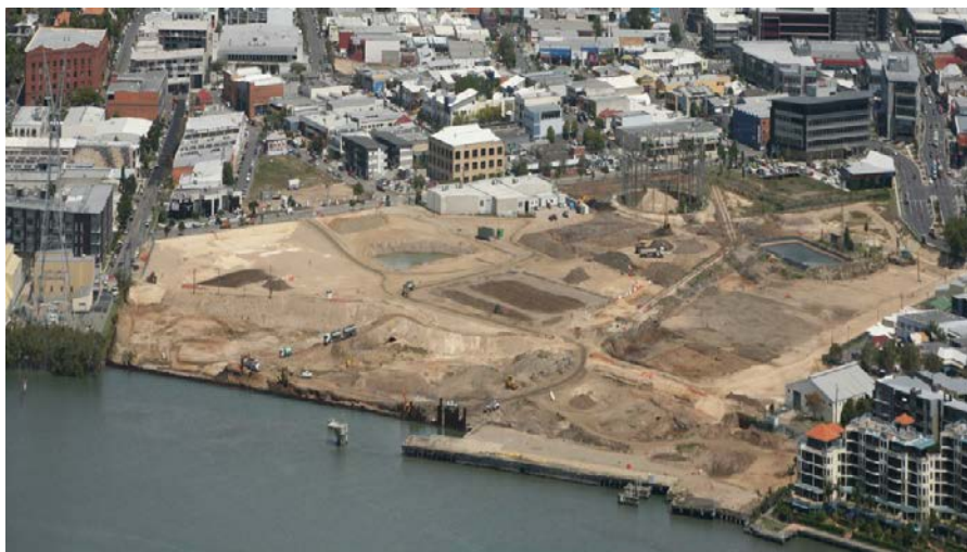
Figure 4.4 Gasworks Newstead Riverpark before Renewal
