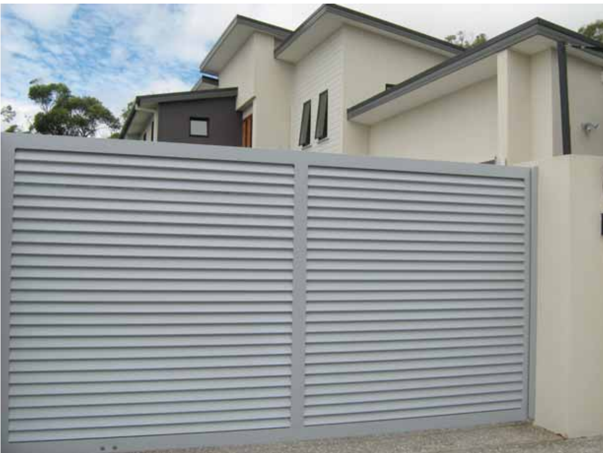
Figure 4.20: An example of a fortified home built in 2008; this is its street face
