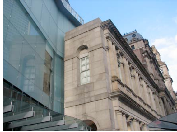
Figure 6. GPO MELBOURNE EXTERIOR (SHOWING NEW EXTENSION)
