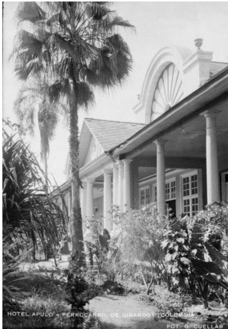
Fig. 4.15 –Hotel Apulo, the centrepiece of the elite’s tropical retreat in Juntas de Apulo
