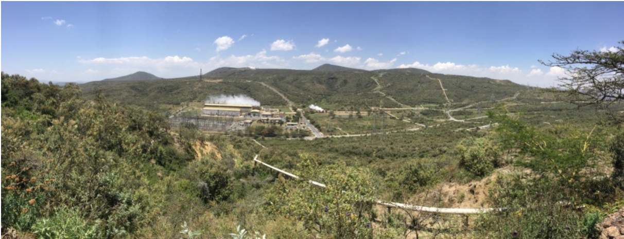
Figure 10. Overview of pipework at power production facilities at the Olkaria Geothermal Field.
