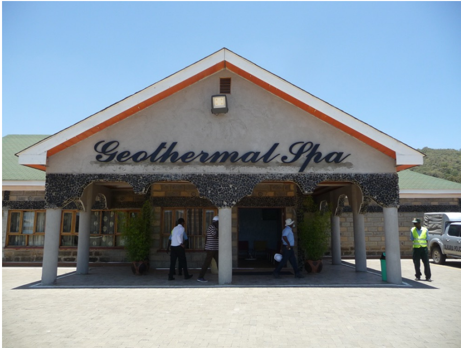
Figure 11. Entrance to the geothermal spa at the Olkaria Geothermal Field.
