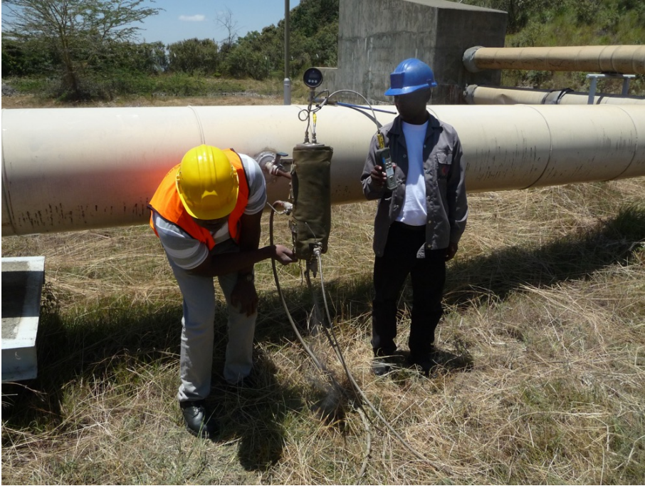
Figure 13. Demonstrating fluid sampling from a pipeline at the Olkaria Geothermal Field.
