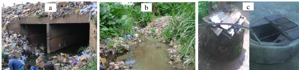
Figure 9.3 Images of waste dumps and blockage of drainage systems (a & b) and unprotected household dug-wells (c).
