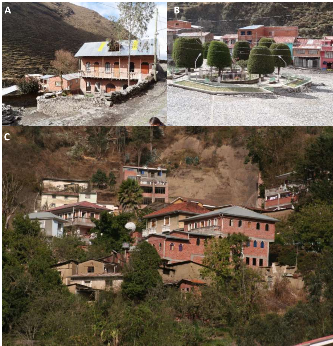
Fig. 5.3. Photos illustrating typical brick structures with roofs made from corrugated steel sheets. Pelechuco (A and B), Sorata (C). Photo credit: Dirk Hoffmann
