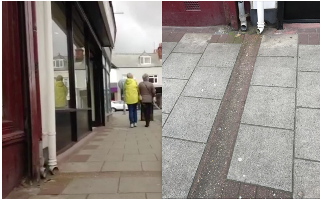
Figure 5: Pavement guttering, likened by C20 to a speed bump (L) view from JourneyCam (R) researcher photo
