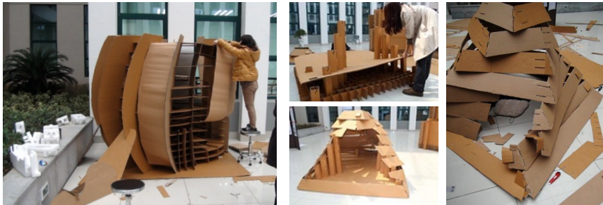
Figure 14. (Left) Using buttresses to transfer extra loads Figure 15. Foundation and inner posts
