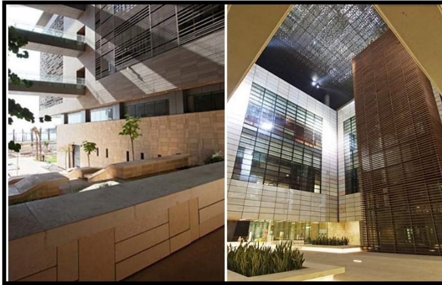
Figure: 6 An interior view of KAUST in Saudi Arabia, which illustrates how to utilise light and shade to enhance the aesthetic value of the building (Meinhold, 2011)
