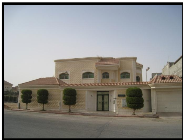
Figure 2: A typical example of a Saudi villa ("Example of a Saudi Villa," 2012)
