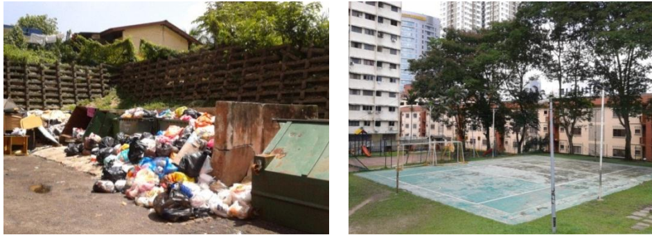
Figure 8: Poor condition of badminton court in KTMB Fla
