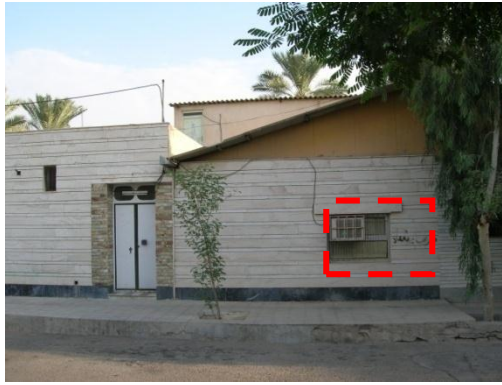
Figure 22: An instance for the applied electrical active air-conditioning system in Lar
