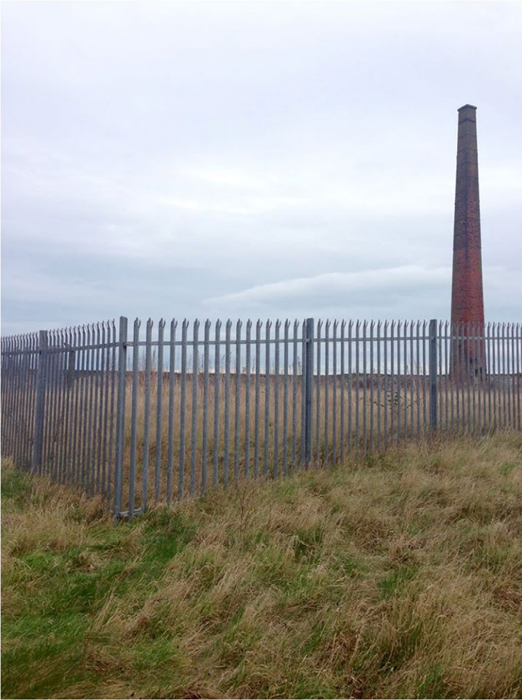
Figure 1: The chimney at Spittal Point. Photo: MG, 2016
